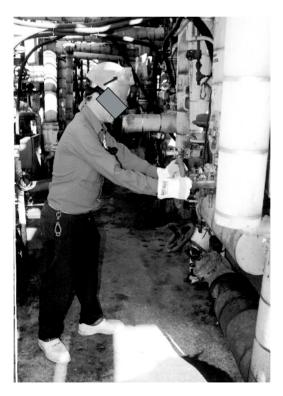
Figure 5-5 Example of good valve stem orientation.
