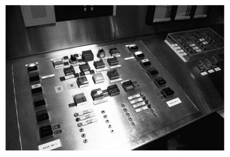
Figure 6-24 Highly reflective stainless steel console is the source of specular glare.
