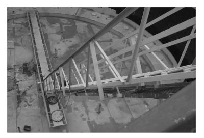
Figure 6-10 Stair ladder installed on a floating roof tank.
