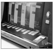
Video Display Terminal (VDT), part of the console located in the control room
