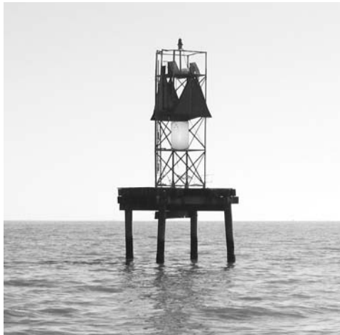
FIGURE 30.5 Modified navigational aid RFID portal.
