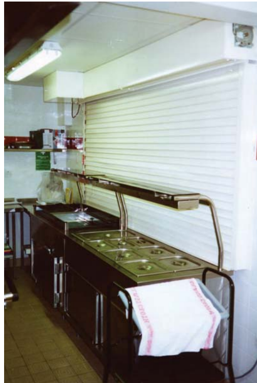
Figure 9.16 Fire shutter
