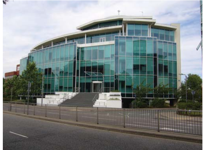
Figure 9.13 Example of a building with an all glass exterior
