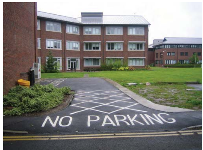
Figure 9.83 Fire service access road
