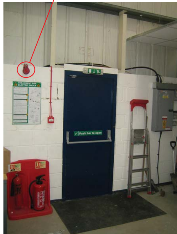
Figure 9.82 An example of a combined audible and visual fire alarm installed in a potentially noisy workplace
