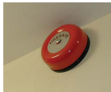
Figure 10.16 Audible warning devices
