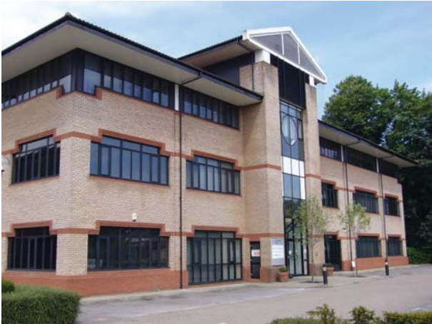
Figure 9.9 Class A – complete non-combustible construction, i.e. concrete or brick floors and walls
