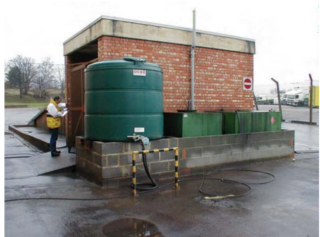
Figure 11.3 Fire safety hazards require active monitoring
