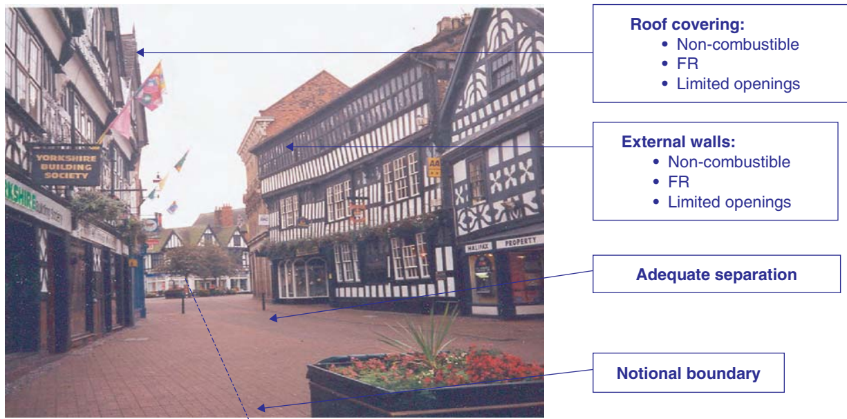
Figure 9.20 Preventing external fire spread
