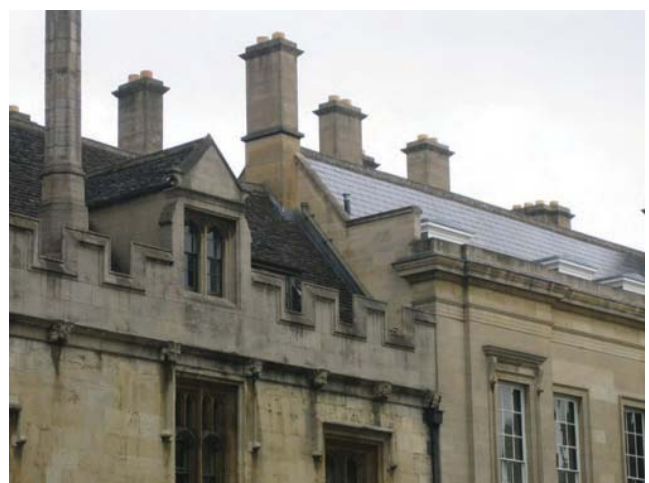
Figure 9.5 Party wall between two adjacent buildings
