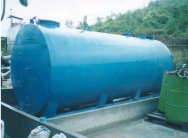
Figure 13.7 Portable tank mounted on a flatbed lorry
