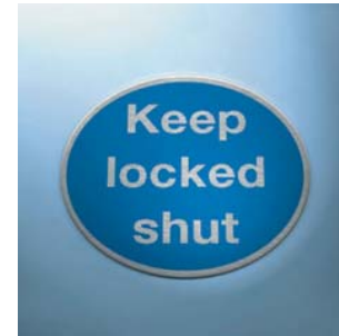
Figure 6.3 Typical fire door keep shut sign
