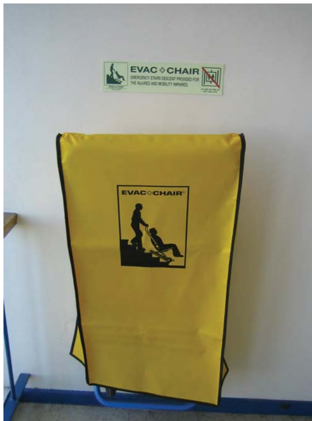
Figure 9.49 Evacuation chair provided to assist non-ambulant persons to escape in case of fire
