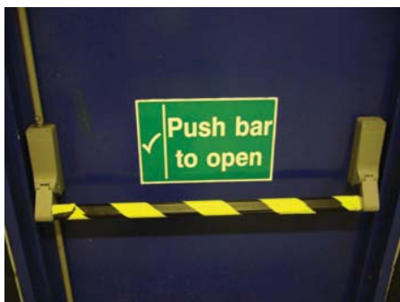
Figure 9.36 An example of a panic device
