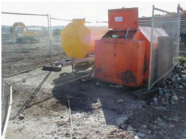
Figure 8.16 External tank facility
