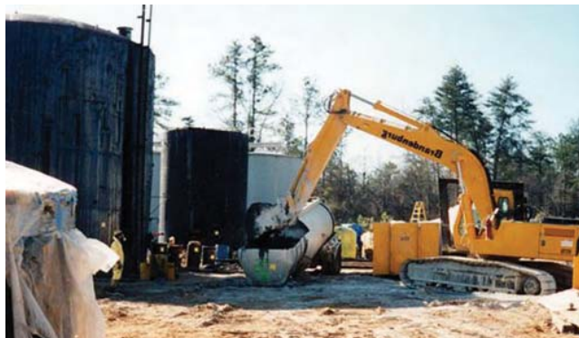
Figure 8.24 Purging tanks during decommissioning
