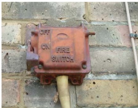
Figure 9.92 Fire fighters switch
