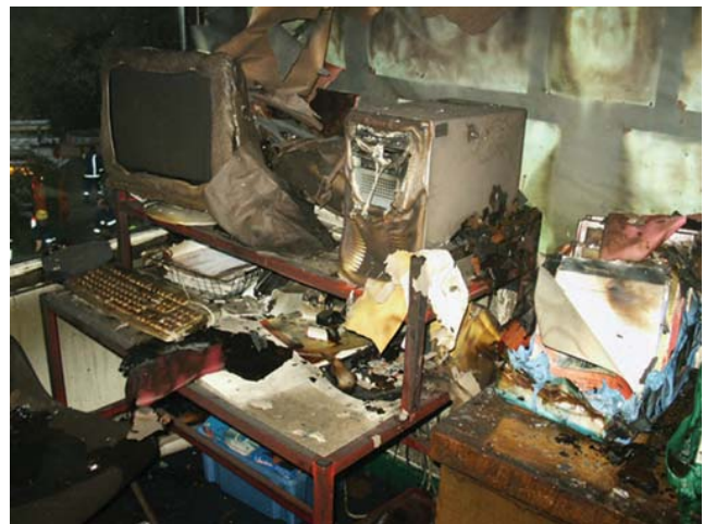
Figure 8.2 Electrical equipment involved in a school fire
