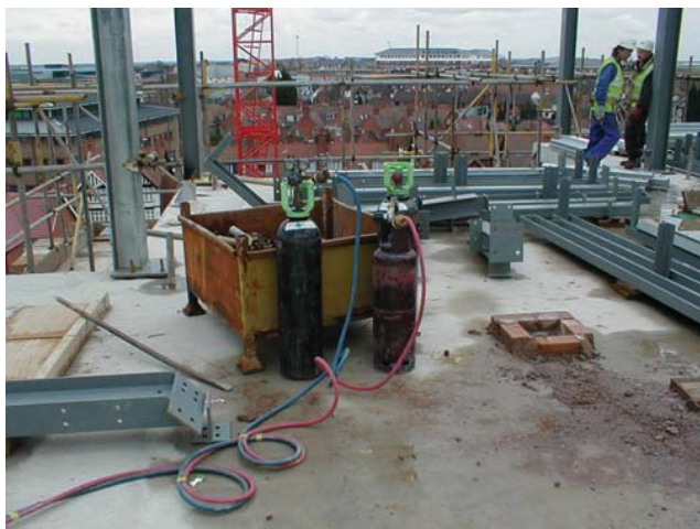
Figure 8.7 Oxy-fuel equipment on a construction site
