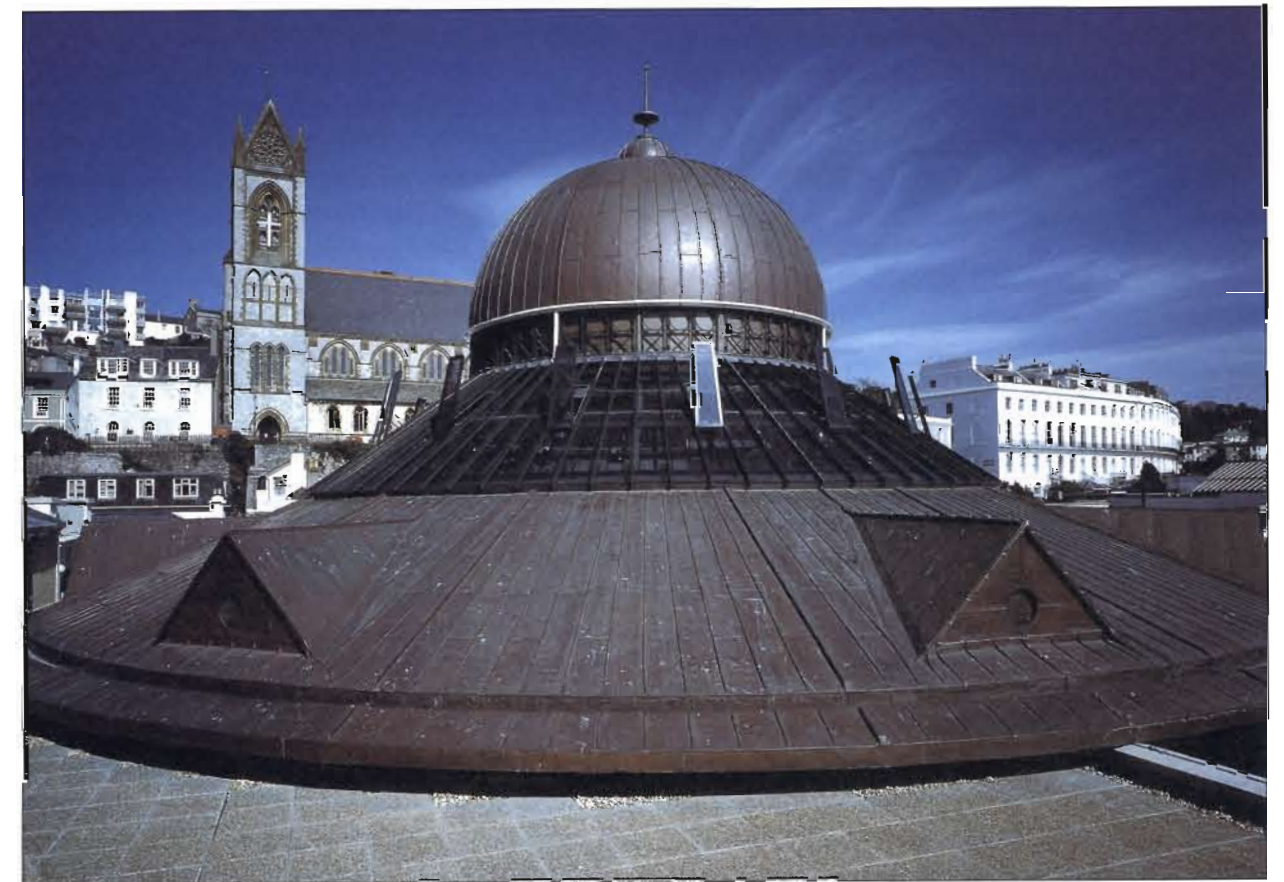
Figure 5.31 An example of metal cladding designed to be a particular feature of a roof. Photo: Broderick Structures.
