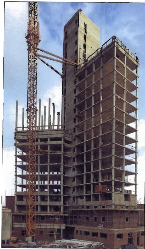
Figure 3.15 Lift-slab construction in its middle stages.
