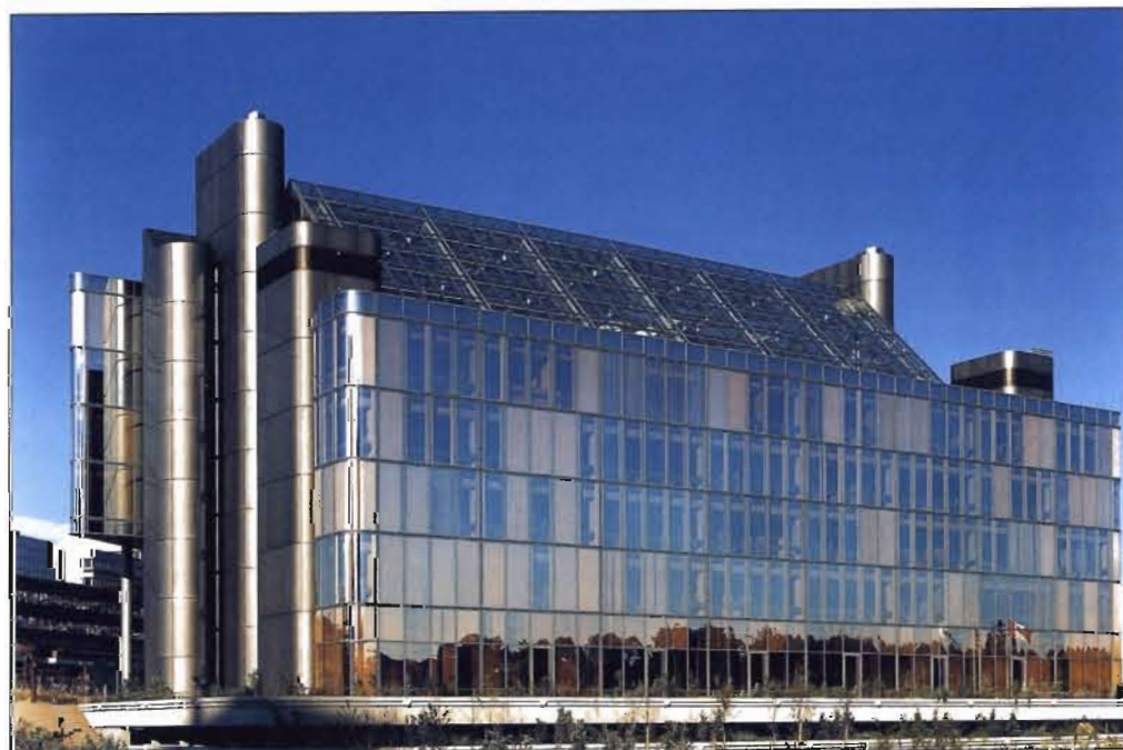
Figure 7.7 Exterior of Figure 7.6 showing almost total glazing with services at each end.
