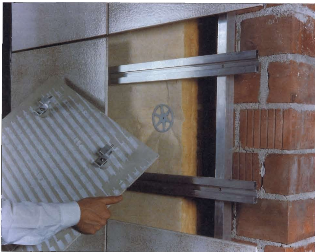
Figure 6.3 A specially designed cladding system fitted to an inner hollowbrick wall.
