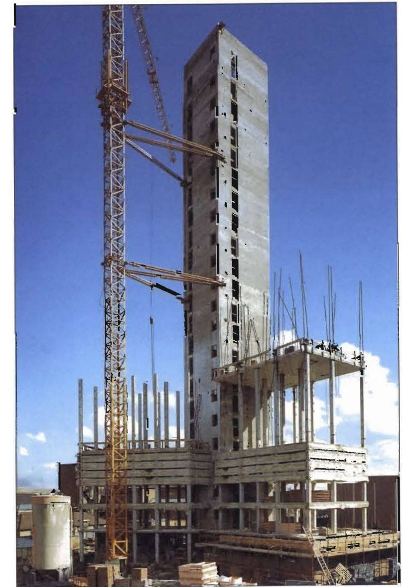
Figure 3.14 Early stage in a lift-slab construction.
