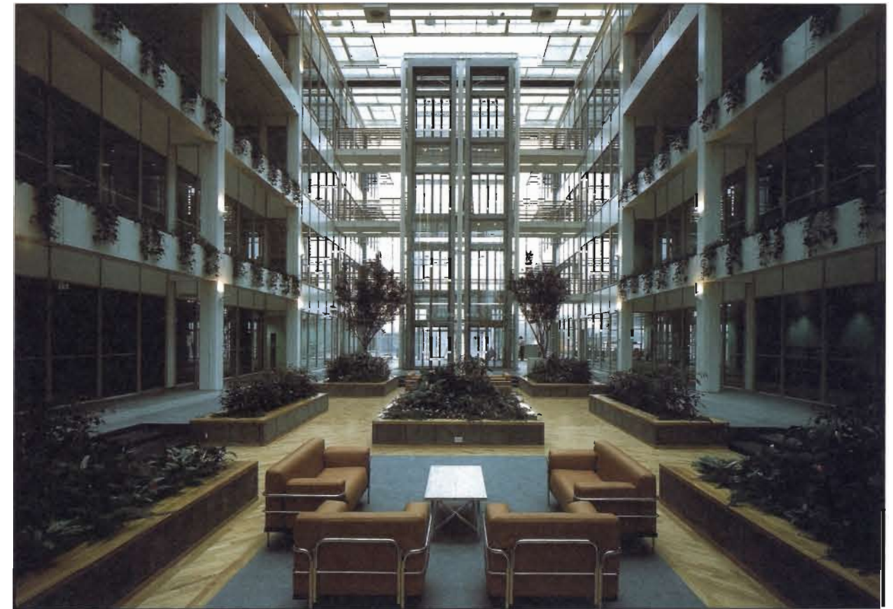
Figure 7.5 Modern office construction with atrium. Fire detectors are visible at second floor level.
