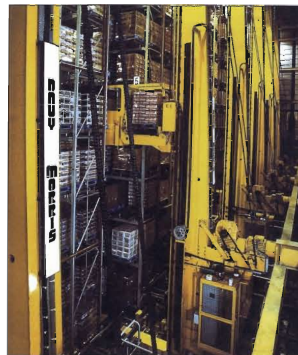
Figure 7.16 The interior of a high-bay warehouse showing automatic picking cranes and the extremely restricted conditions in the racking area. Photo: Rowntrees Mackintosh.
