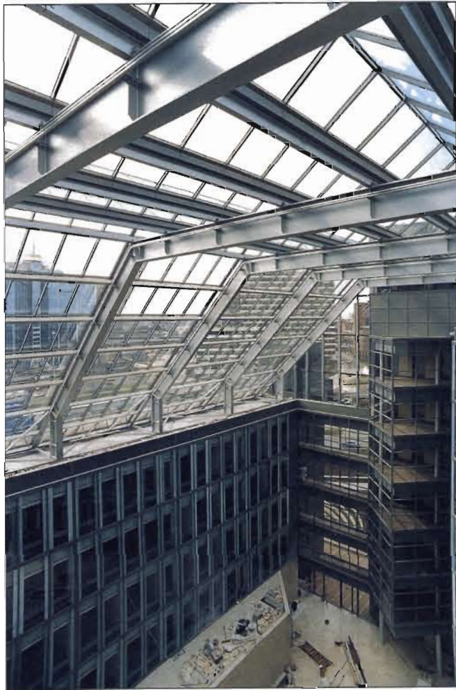
Figure 7.6 Interior of offices under construction (see Figure 7.7).
