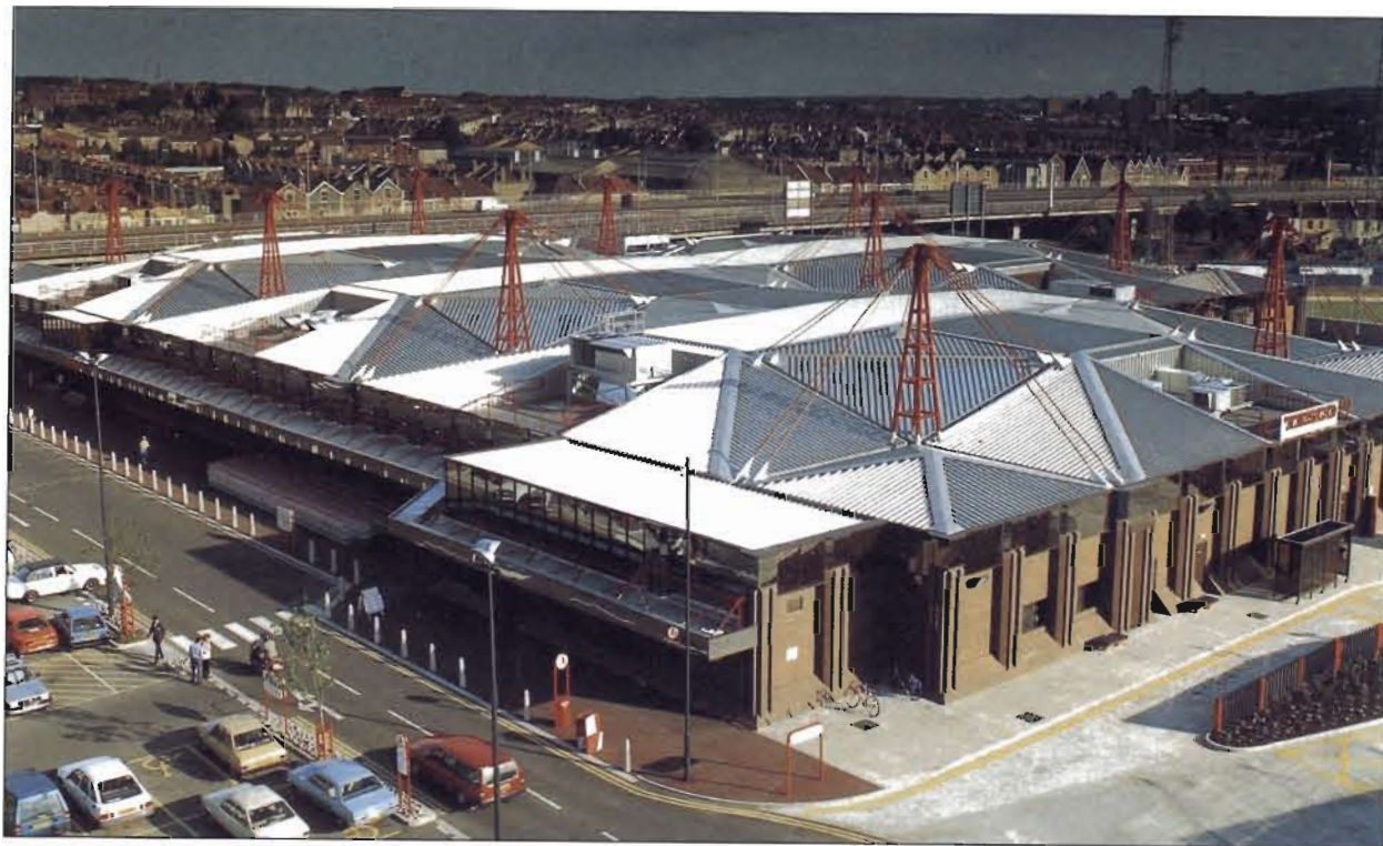
Figure 3.6 A supermarket showing the method of suspended roof support. Photo: Ernest Ireland Construction.
