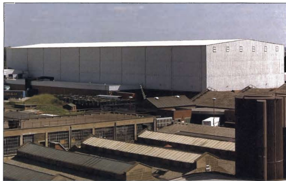
Figure 7.15 A high-bay warehouse 155m x 55m x 22m, totally enclosed. The six large smoke outlets are repeated at the other end. Photo: Rowntrees Mackintosh.
