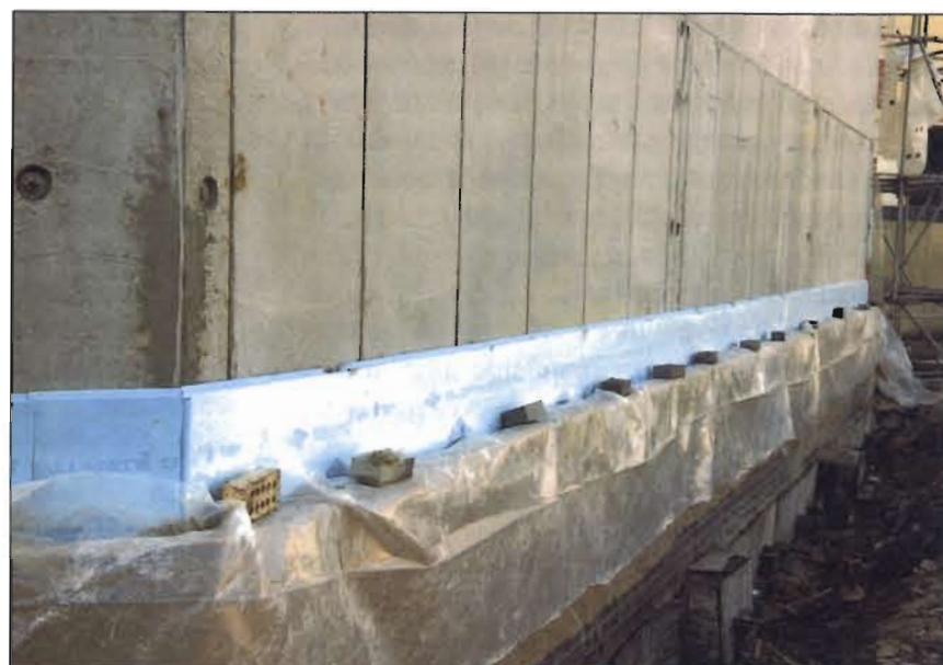
Figure 6.2 Polystyrene insulating sheeting placed between the inner wall and the brick cladding.
