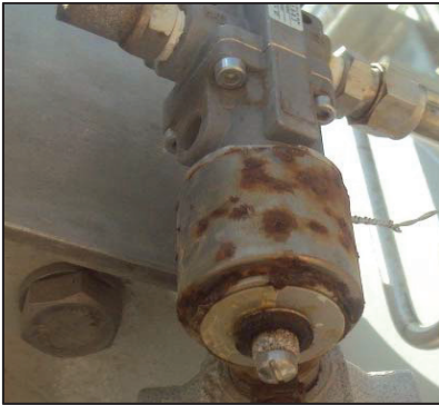
Figure 8.1. Corroded Solenoid
