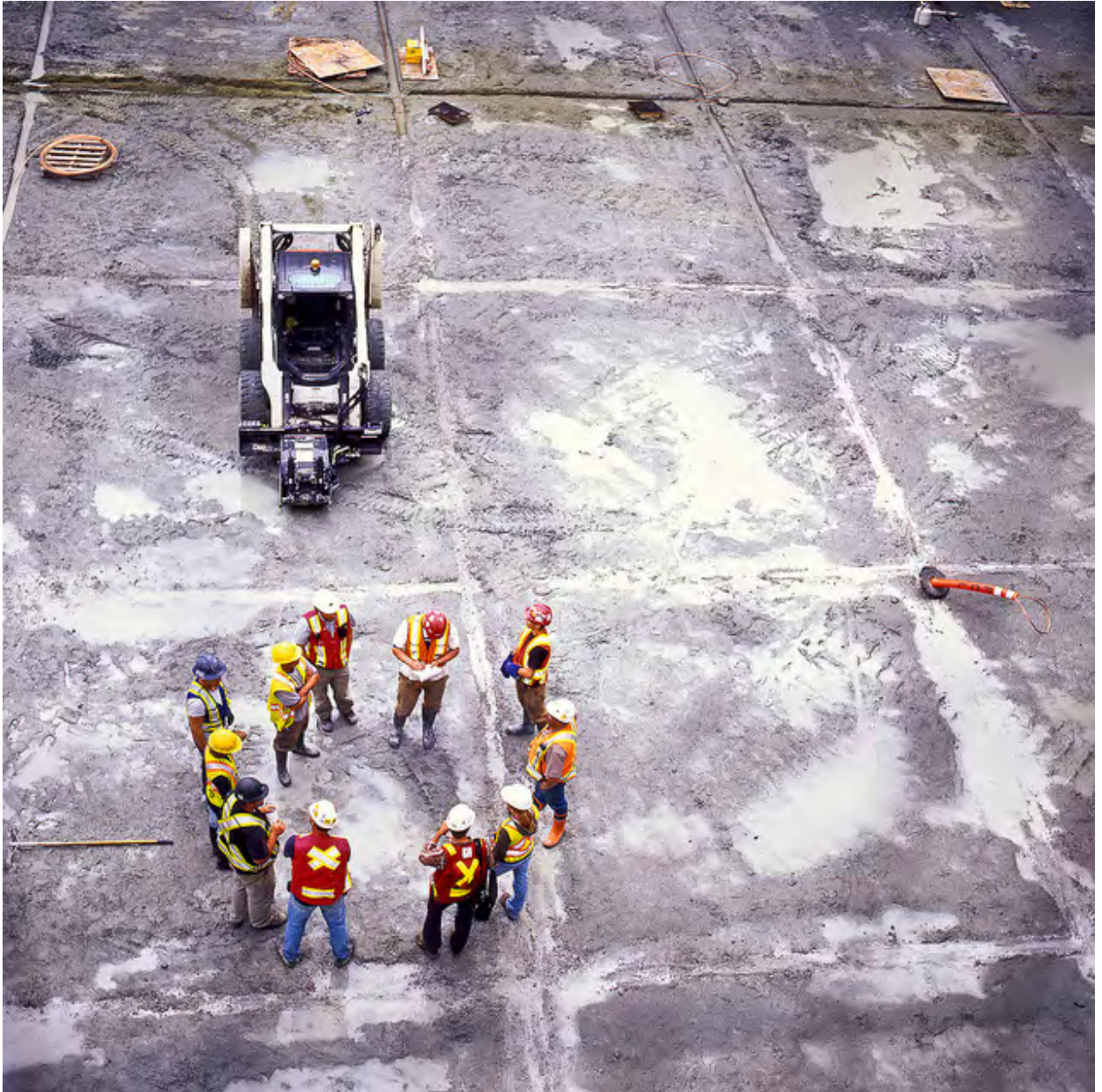
Figure 13-1: Construction crew performing PTP (Picture Courtesy Guy F. Atkinson Construction)
