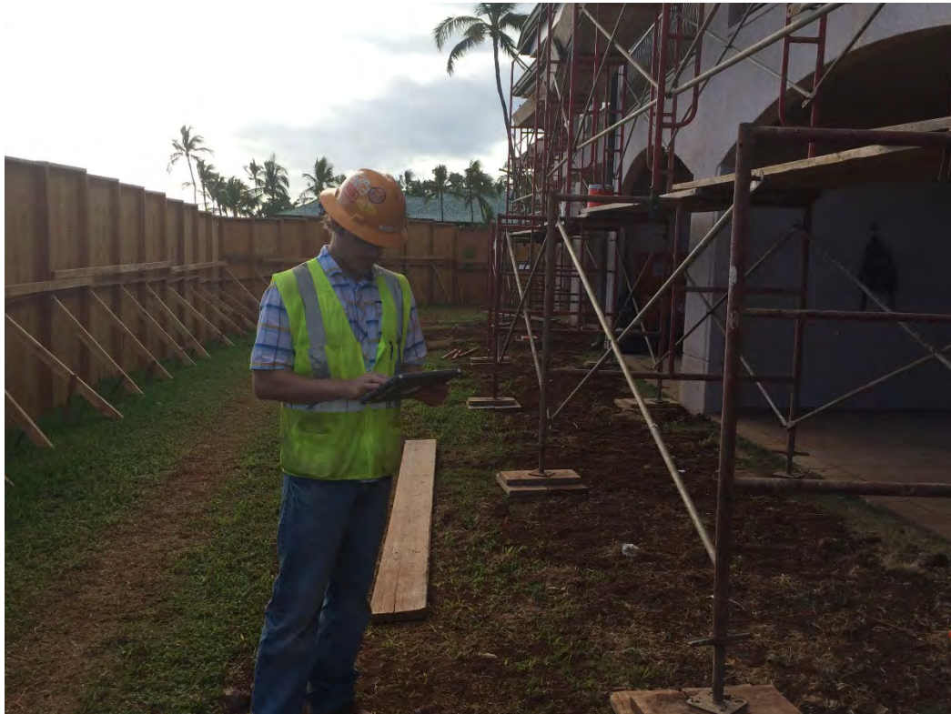
Figure 21-1: Safety Professional Performing Scaffold Inspections using I-pad (Courtesy Hensel Phelps Construction)
