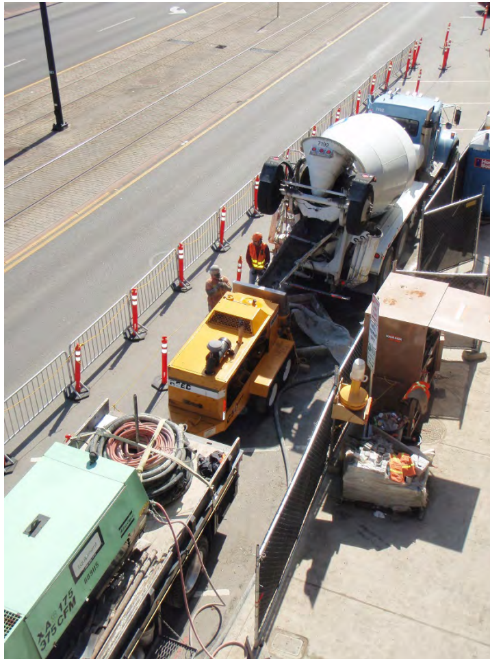
Figure 10-5: Example of Traffic Control around Construction Sites (Picture Courtesy of Korsmo Construction)
