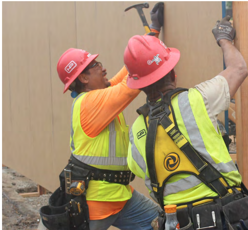
Figure 10-3: Workers Installing Project Perimeter Privacy Barricade (Courtesy of Hensel Phelps Construction)
