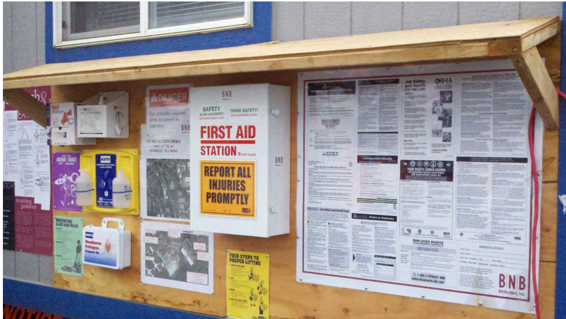
Figure 9-2: Example Safety Station/Bulletin Board with weather protection (Picture Courtesy BNBuilders)
