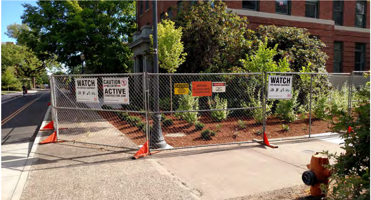
Figure 10-2: Example of Properly Installed Site Fence with Appropriate Warning Signage (Picture Courtesy of Hoffman Construction Company of Oregon).
