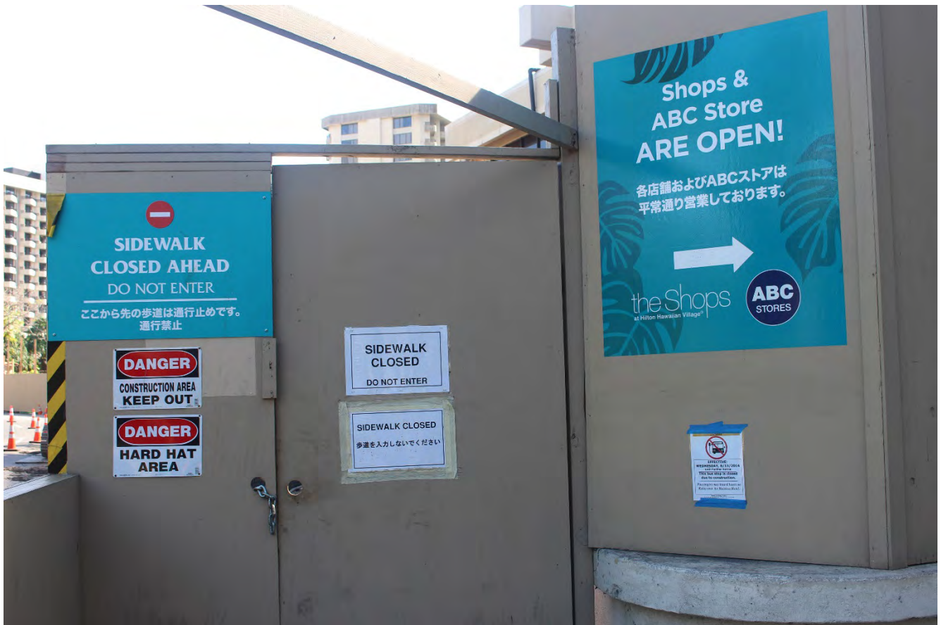
Figure 10-7: Example of Sidewalk Closed Signage and Barricade (Picture Courtesy of Hensel Phelps Construction)
