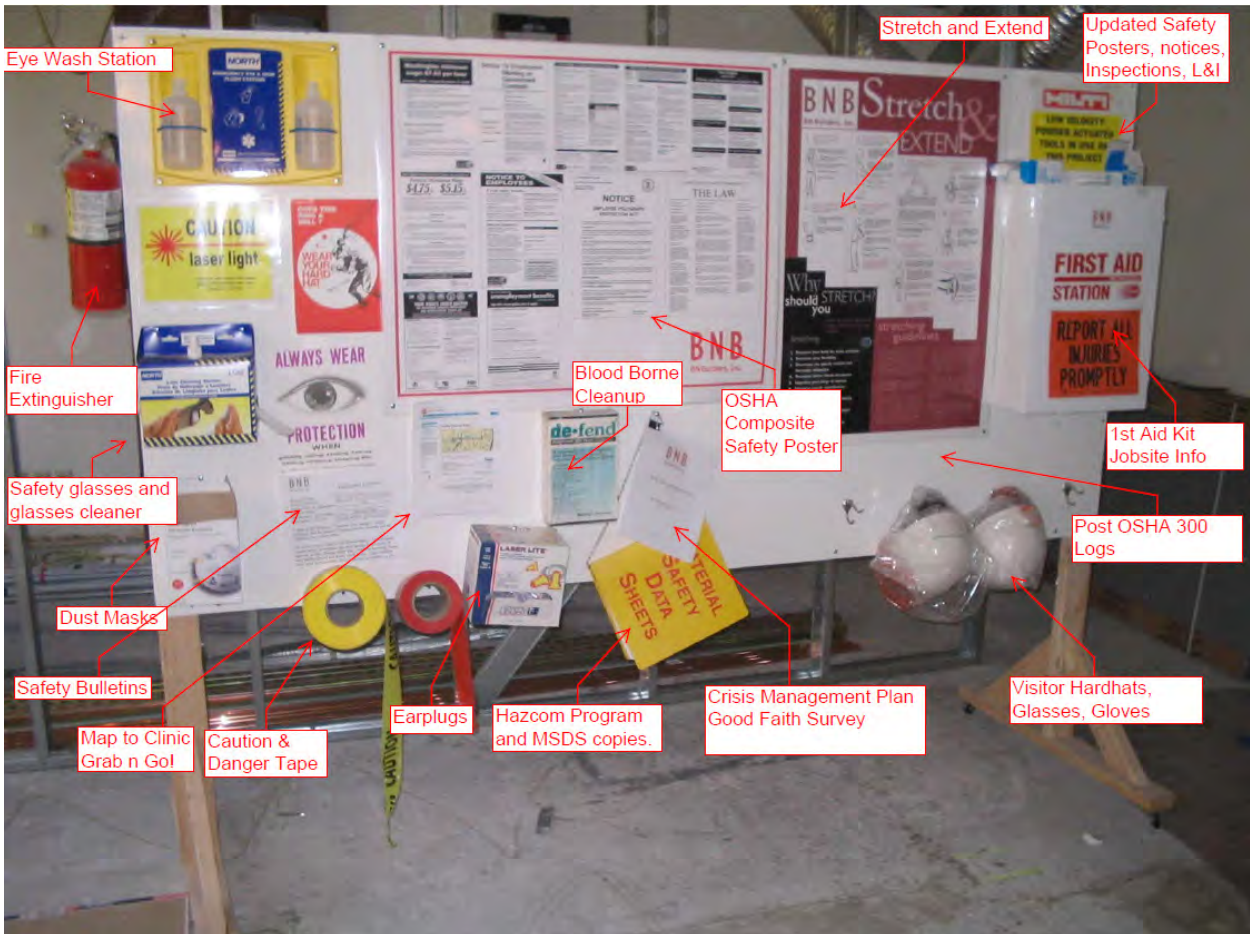
Figure 9-1: Example Safety Bulletin Board (Picture Courtesy BNBuilders)
