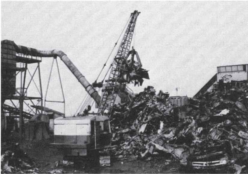
Plate 1. A fragmentation plant for efficient breaking down of scrap cars into their constituent materials—ferrous and non-ferrous metals, plastic, etc. Such a plant can be a serious noise problem to nearby residents
