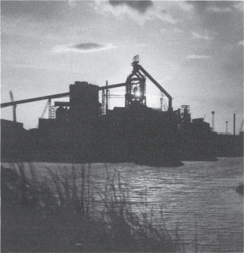
Plate 1. Large plant can produce significant environmental noise problems.
