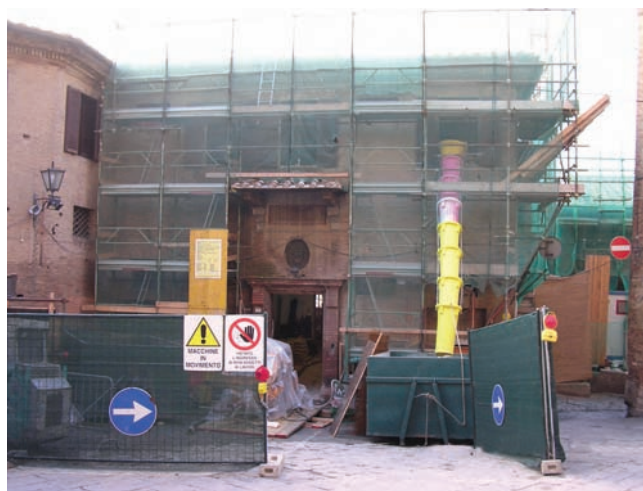
Figure 18.9 Construction site – Sienna.
