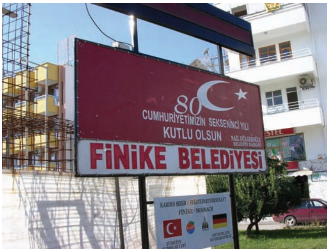
Figure 18.2 Local authority building site, Turkey.
