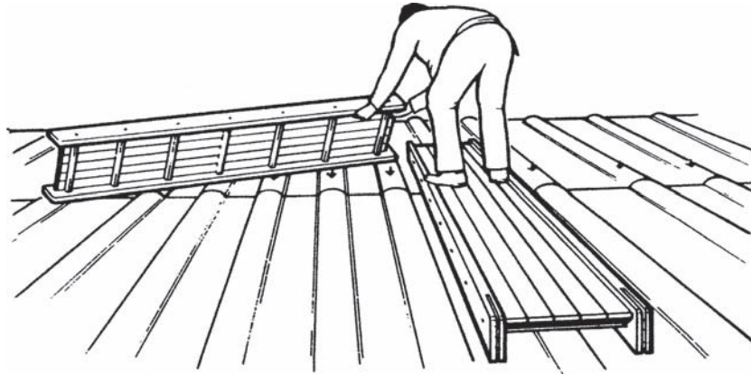
Figure 16.2 Proper precautions must always be taken when working on or near fragile roofs.
