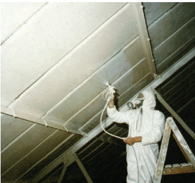
Figure 5.4 A lone worker – special arrangements are required.
