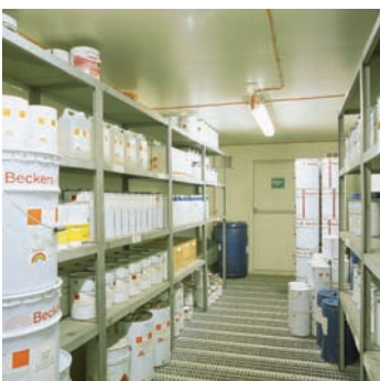
Figure 13.8 Various storage arrangement for highly flammable liquids.
