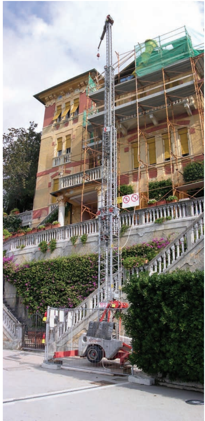
Figure 18.12 Mobile tower crane – Cinque Terre, Italy.
