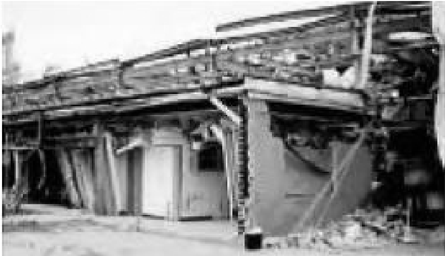
Figure 3.26. Damage to Flixborough control room.
