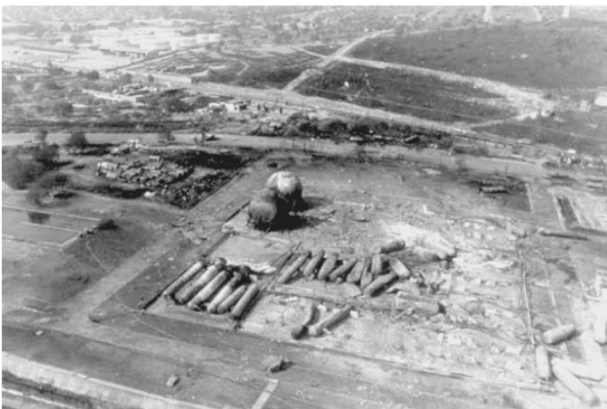
Figure 3.35. PEMEX LPG Terminal after the explosion source, CCPS, 2008.
