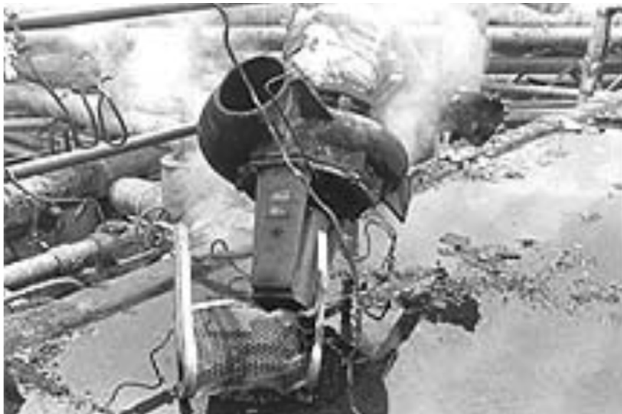
Figure 5.2. Pump explosion from running isolated.
