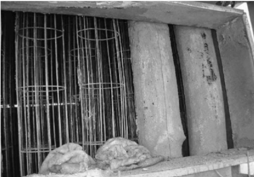
Figure 5.15. Damage to dust collector bags, Ref. 5.25
