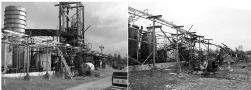
Figure 5.22. T2 Laboratories site before and after the explosion, Ref. 5.28.
