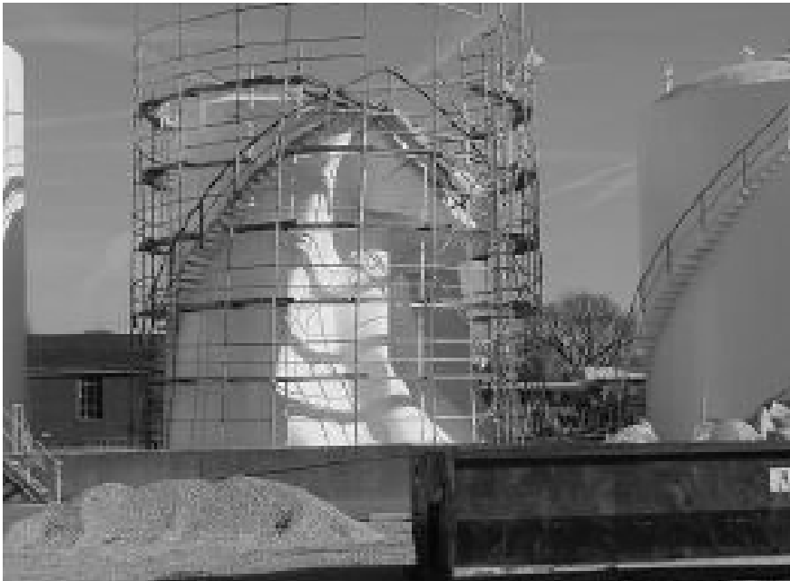
Figure 5.32. Tank collapsed by vacuum.
