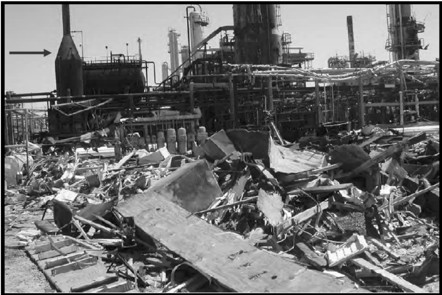
Figure 3.4. Portable buildings destroyed where contractors were located, courtesy CSB.
