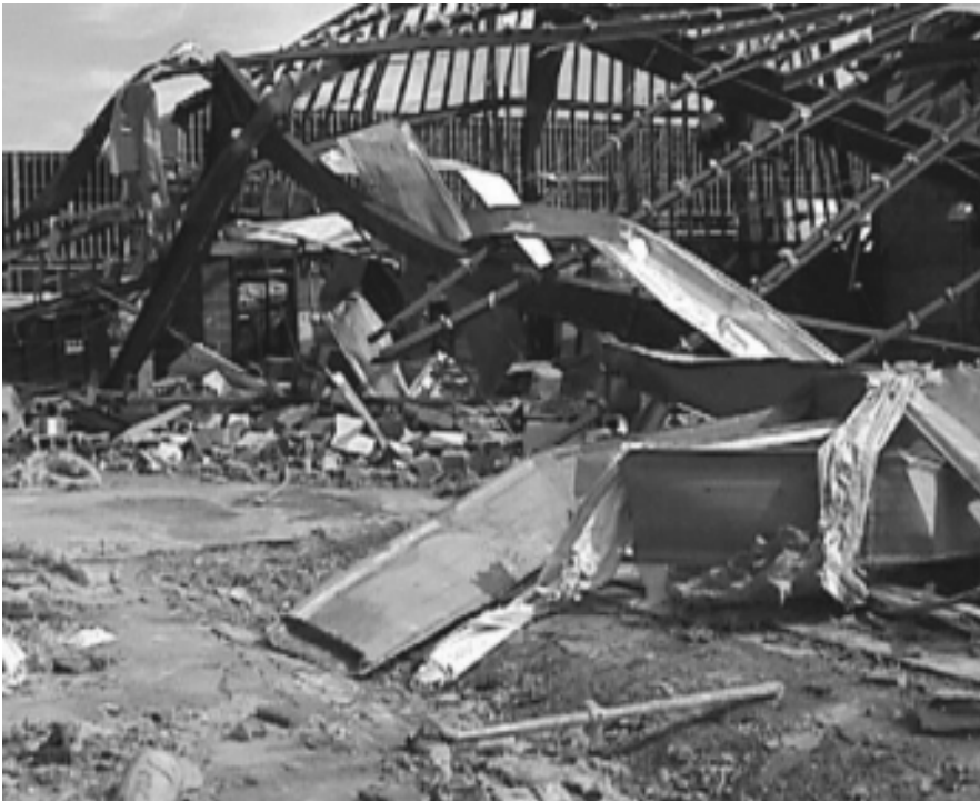
Figure 2.5. Building damage and charge tank crater, Hydroxylamine explosion, courtesy CSB.
