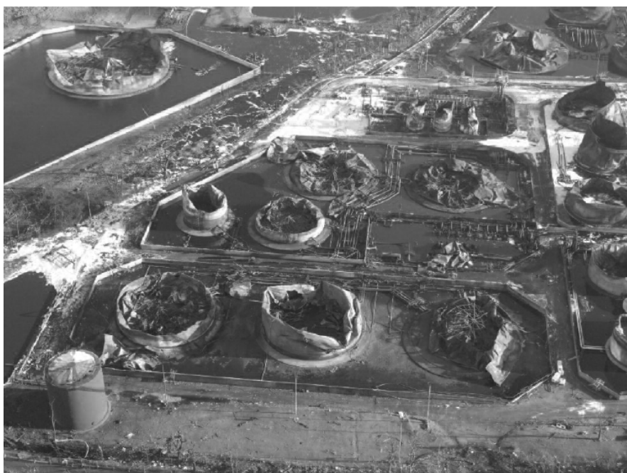
Figure 5.28. Buncefield after the explosion and fires, Ref 5.32.
