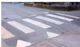
Figure 17 This pedestrian crossing has been combined with a well-marked speed hump
