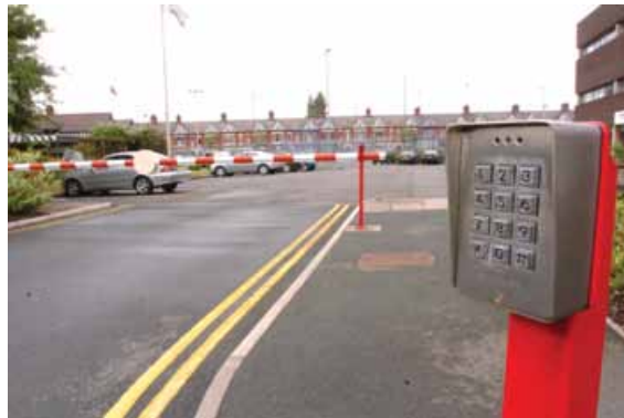
Figure 2 Key pad accessible from driving position
