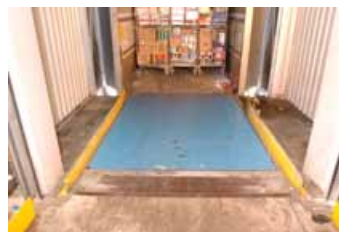
Figure 31 An extended dock leveller linking a loading bay to a vehicle load body
