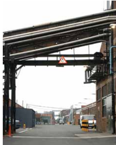
Figure 4 This overhead structure is signposted with a height restriction
