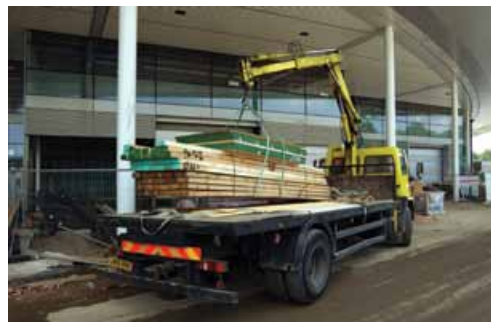
Figure 49 Vehicle unloading from firm and level ground
