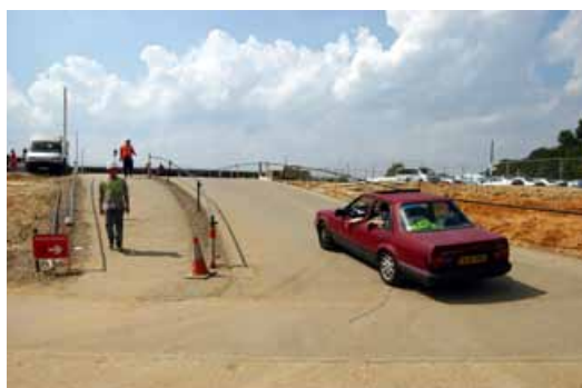
Figure 30 Pedestrians are segregated from vehicles on this slope
