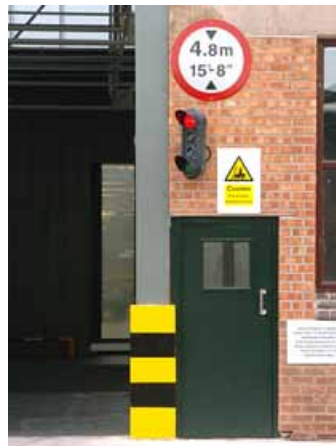
Figure 9 This well-organised building entrance separates vehicles and pedestrians as well as being clearly marked and providing signals and signs for drivers
