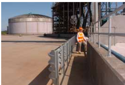
Figure 16 Barrier to protect pedestrians
