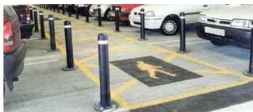
Figure 27 Pedestrian walkway in car park
