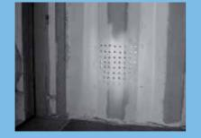
Make 4 to 8 rodent proof lower lateral 12" x 12" air vents by drilling series of 1/2" holes through the inner groove of the container wall. (Inside view)
