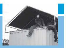
Build a roof (canopy structure, tin roofing, ...) preferable with an angle of 120° and fix it to the container.
