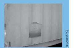
Cover these air vents on the outside with home made moulded galvanized steel plates welded 3/4 around to prevent vertical & lateral water infiltration.
