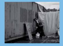
Place the container on 10" reinforced concrete blocks. repair it where necessary and make it weather and rust proof (1 inch = 2.5 cm).
