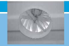
Cut out the opening for the turbine ventilator and weld a (4") inch circular turbine base to the opening. (The base must not stick out more than (2") inches).
