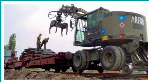
Engineer crane at work
