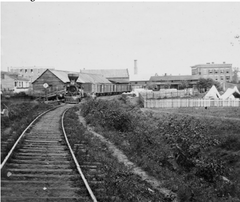
4.3. Freight Train at Culpeper Courthouse, Virginia. This photograph was exposed by Timothy H. O'Sullivan in August 1862. Grass and weeds grow on the railroad bed in this view, coming close to topping the rails. If that happened, it could lessen the friction needed for the iron wheels to grip the rails, slowing or even stopping a train. One can see an engine and about a dozen cars occupying a siding. (Library of Congress, LC-DIG-cwpb-01078)
