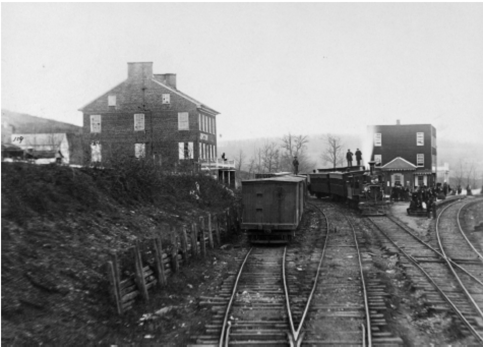
4.6. Railroad Junction at Hanover, Pennsylvania, August 1863. Two lines served Hanover Junction, the Hanover Branch Railroad and the Northern Central Railroad. One line, on the left, has two sidings, but the other line on the right has none. An engine, boxcars, and passenger cars are visible in this view and the building on the right still stands today, housing a railroad museum. The tall man wearing a stovepipe hat in front of the building has been thought to be Abraham Lincoln on his way to Gettysburg on November 18, 1863, but the original label in the Library of Congress indicates the photograph was exposed the previous August. (Library of Congress, LC-DIG-ppmsca-35054)
