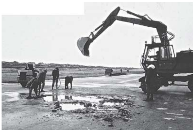
Although bombs and shells never succeeded in stopping Argentine cargo planes from landing at Stanley, they had created damage needing repair before British C-130s from Ascension Island would land. Here engineers start repairing the airfield. The first
