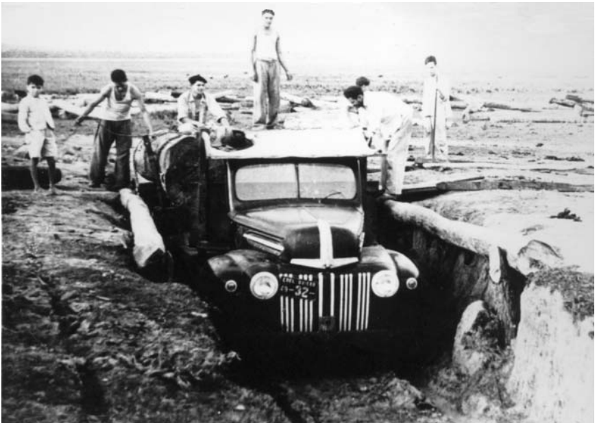
Figure 3-1 Truck loading-unloading facility achieved by digging a hole to place truck bed at ground level. Photo courtesy of Organization of American States, Columbus Memorial Library, Photograph Collection.
