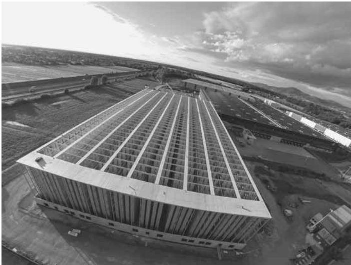
FIGURE 9.6 Alnatura distribution centre in Lorsch, Germany (under construction)
