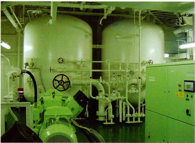
▲ The air receivers for a large two-stroke crosshead engine – Category IV.
