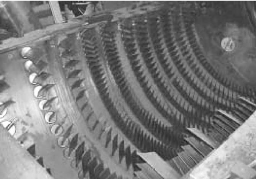
Figure 7-3. Axial-flow compressor stators located in the casing.
