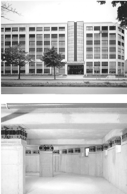
Figure 1 Typical base-isolated building in the form of a multistory office. (Courtesy of GERB Schwingungsisolierungen GmbH & Co, Germany.) The entire building is isolated from its foundation by spring bearings located in the basement.
