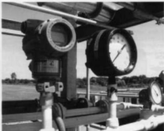
**FIGURE 12.18** Pressure transmitter (left) and pressure gage (right).
