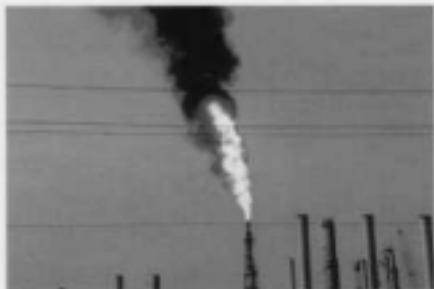
**FIGURE 20.4** Typical elevated single-point flare.
