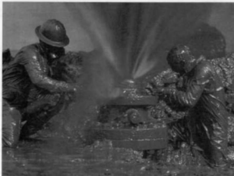
**FIGURE 5.36** Capping a burning oil well.
