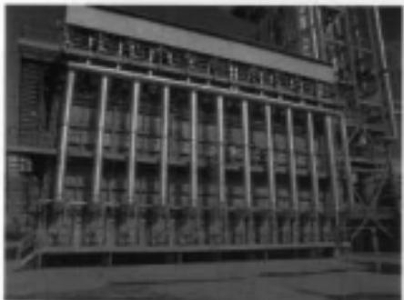
**FIGURE 15.7** Burners mounted on the side of a heater.
