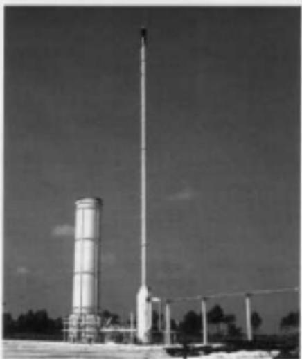
**FIGURE 20.9** Combination ZTOF and elevated flare system.
