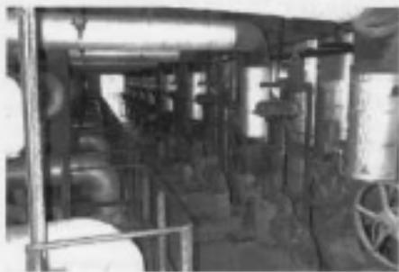
**FIGURE 15.9** Burner mounted in a common plenum.
