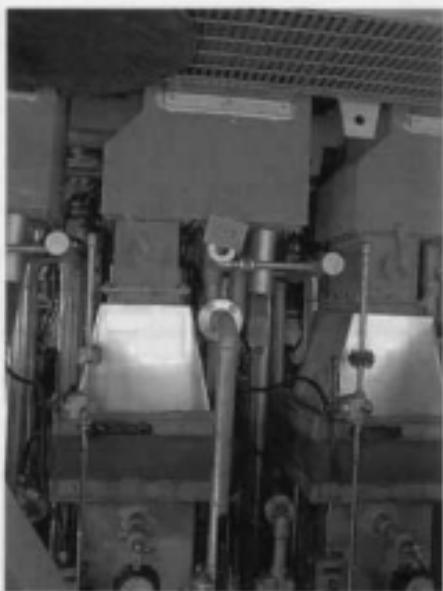
**FIGURE 15.8** Burner mounted on the top of a heater.
