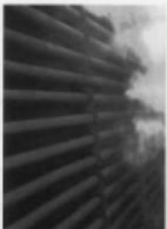
**FIGURE 1.40** Flames impinging on tubes in a cabin heater.
