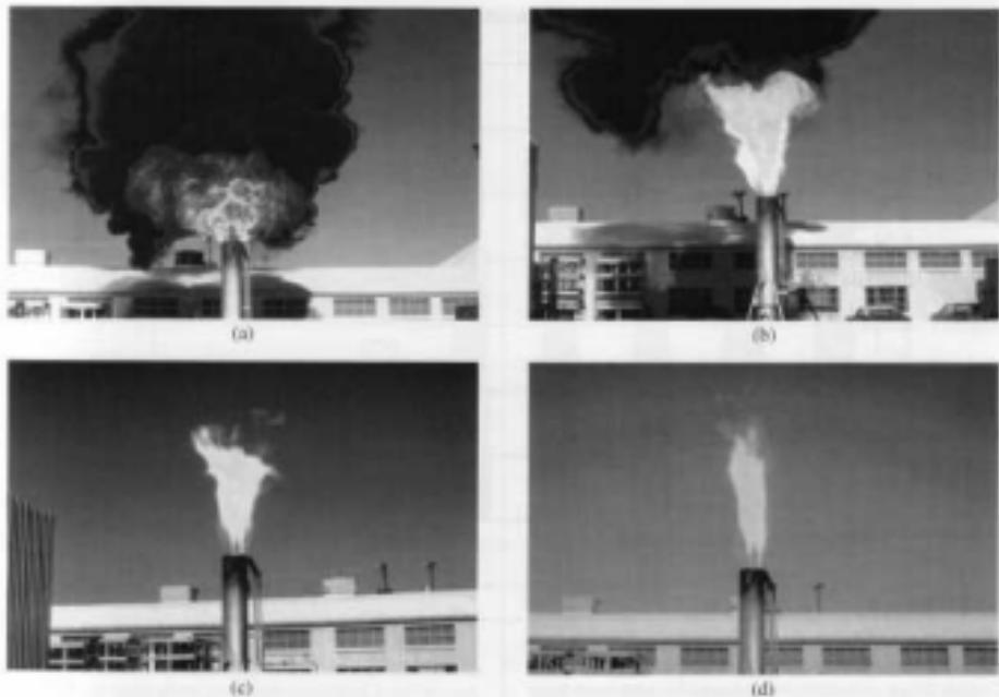
**FIGURE 20.19** Effectiveness of air in smoke suppression: (a) no blower air, (b) start blower, (c) air flow increasing, and (d) smokeless.
