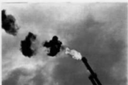
**FIGURE 20.45** "Smoke signals" from a surging liquid seal.
