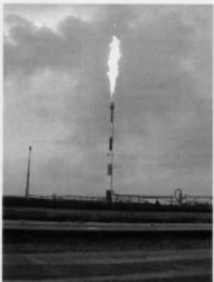
**FIGURE 8.24** Smokeless steam flare designed with new method.
