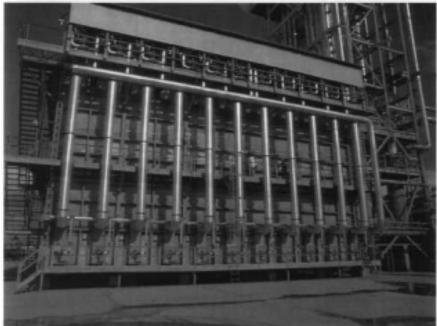
FIGURE 15.20 Typical fuel gas piping system.
