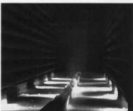
FIGURE 1.15 Horizontal floor-fired burners.
