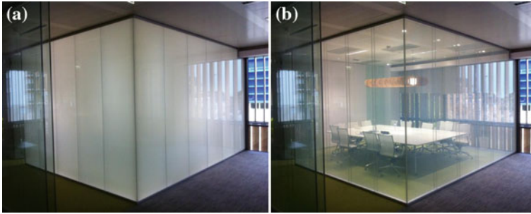
Fig. 5.14 Subdivision inside the Microsoft Head Office, Lisbon in the switched off ( left ) and switched on modes ( right ). Courtesy SmartGlass International
