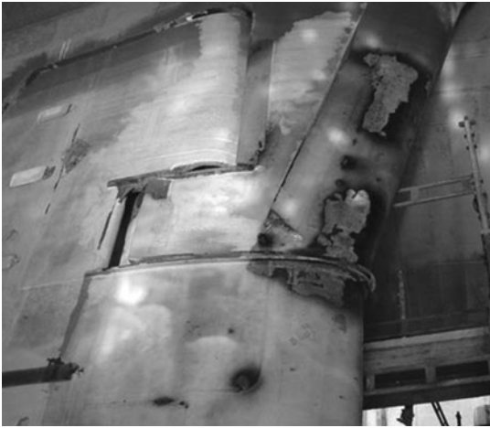
Figure 9.39 Example of rudder erosion
