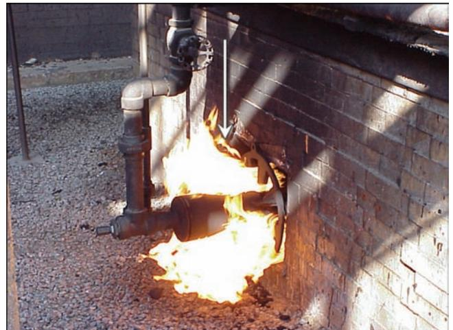
**FIGURE 9.57** Positive draft inside a heater forcing flame out through the burner intake.
