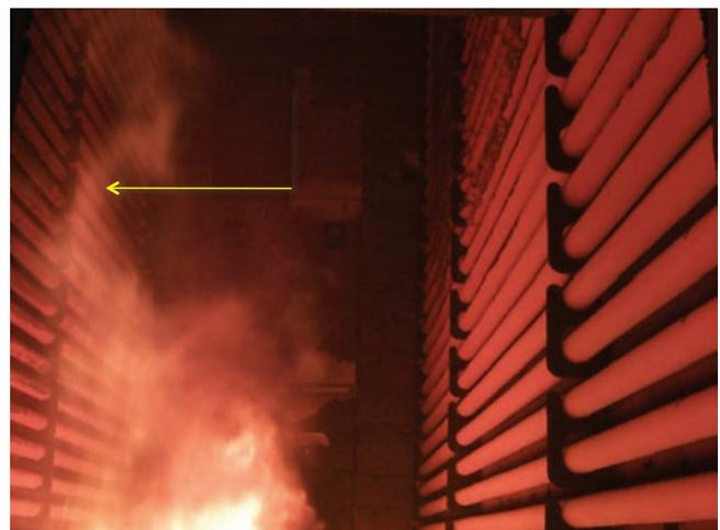
**FIGURE 9.124** Flames impinging on process tubes in radiant section.
