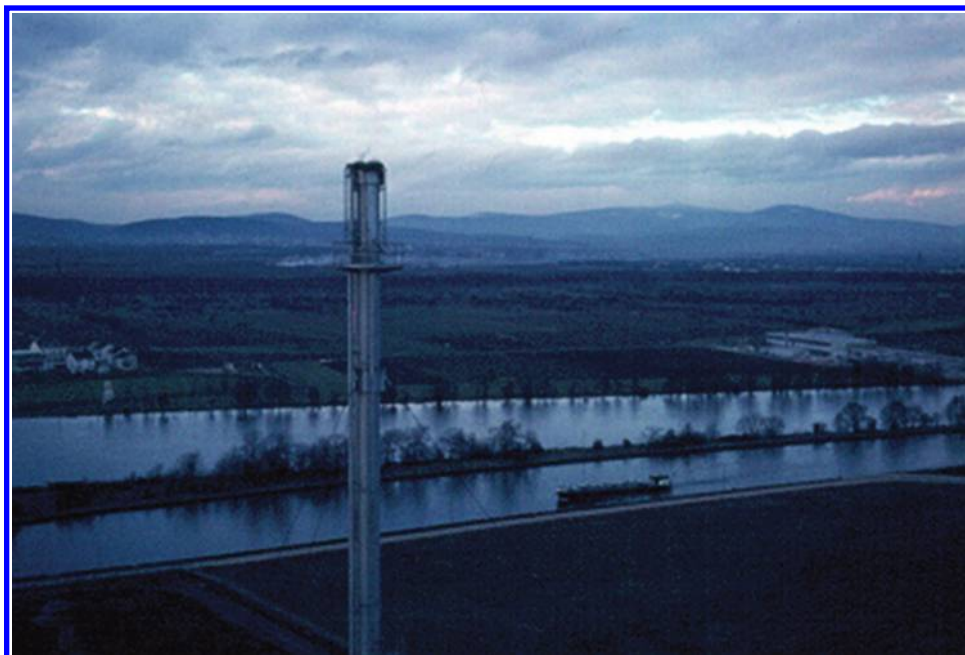
FIGURE 11.23 Simple steam-assisted flare.
