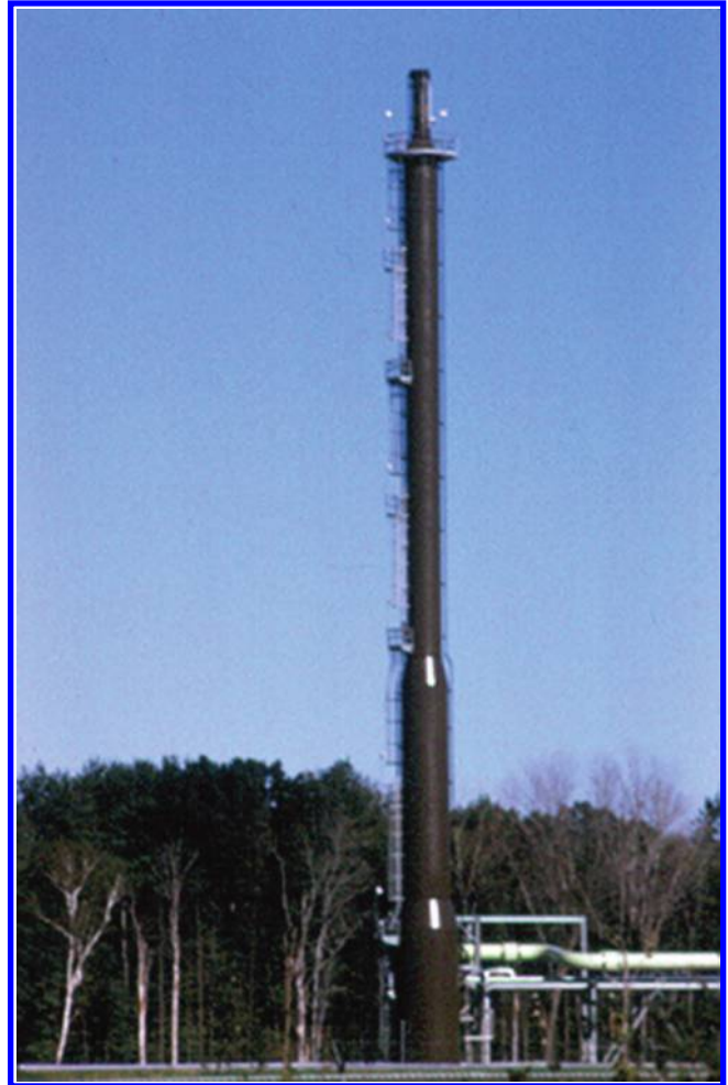
FIGURE 11.46 Self-supported flare.
