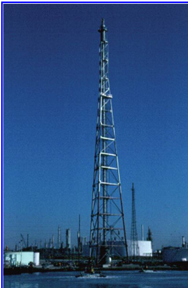
FIGURE 11.48 Derrick-supported flare.
