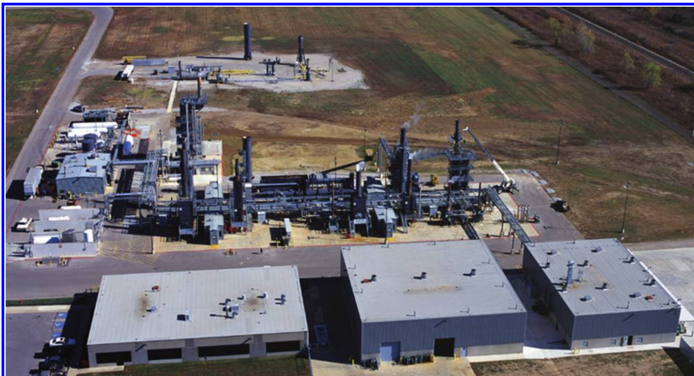
FIGURE P.3 Flare testing facility.
