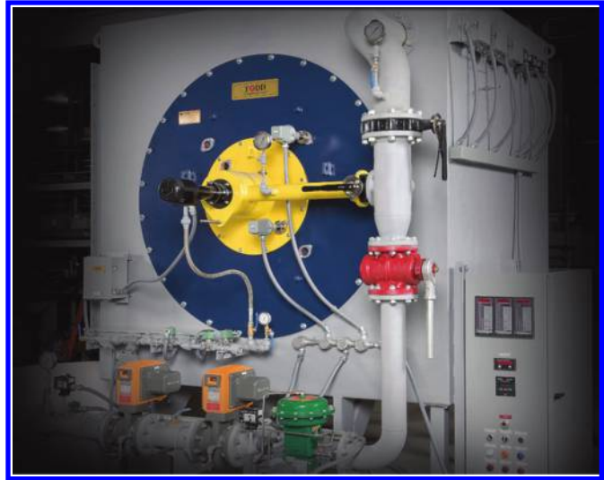
FIGURE 3.17 Coen D-RMB ® burner mounted inside the wind box.
