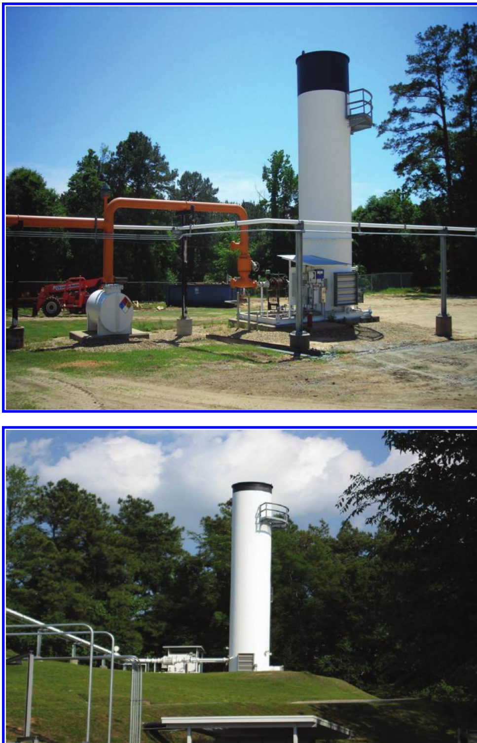
FIGURE 15.15 Photos of vapor combustors.
