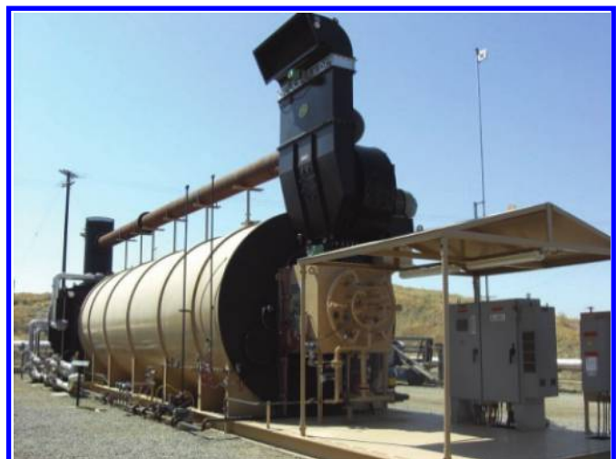
FIGURE 3.28 Row of boilers equipped with Coen QLN-II™ burners rated to 63 and 90 × 10 6 Btu/h (18.5–26 MWt).
