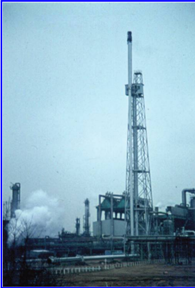
FIGURE 11.49 Demountable derrick.
