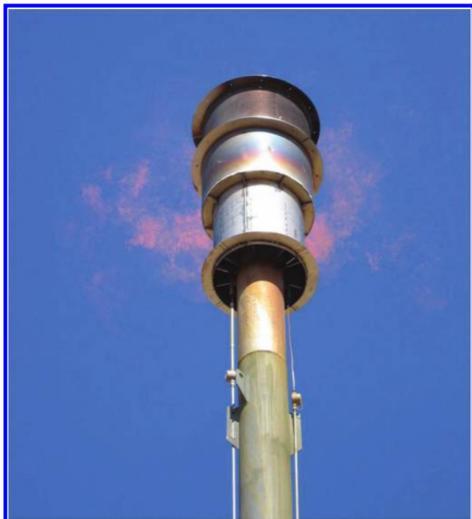
FIGURE 13.3 Unconfined flame extending beyond the windshield.
