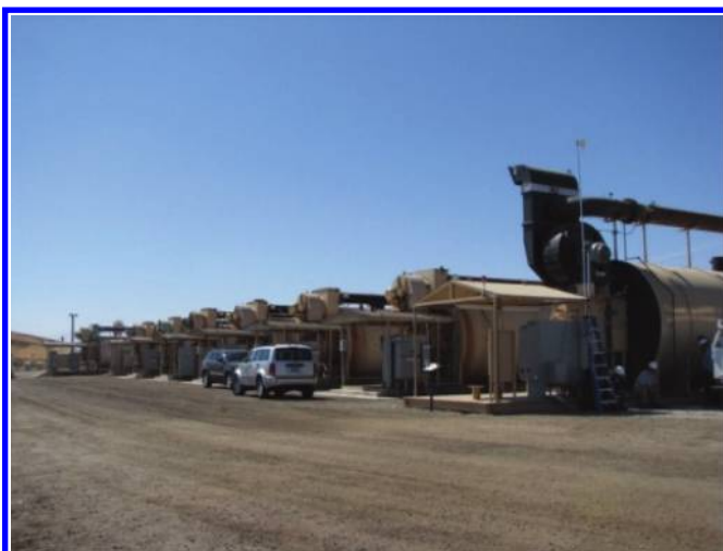
FIGURE 3.28 Row of boilers equipped with Coen QLN-II™ burners rated to 63 and 90 × 10 6 Btu/h (18.5–26 MWt).
