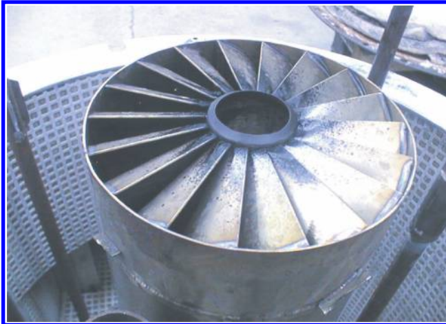
FIGURE 2.14 Swirler for oil firing on forced draft.
