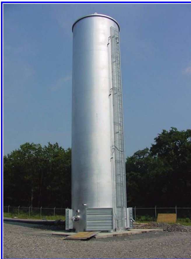
FIGURE 13.4 Enclosed flare.
