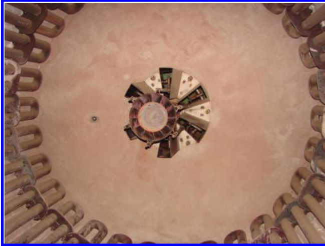
FIGURE 3.27 Coen QLN-II burner inside a furnace.
