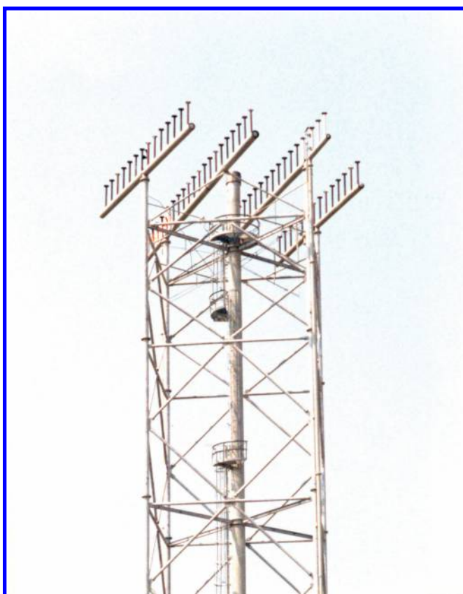
FIGURE 11.10 Combination elevated LRGO and utility flare system.
