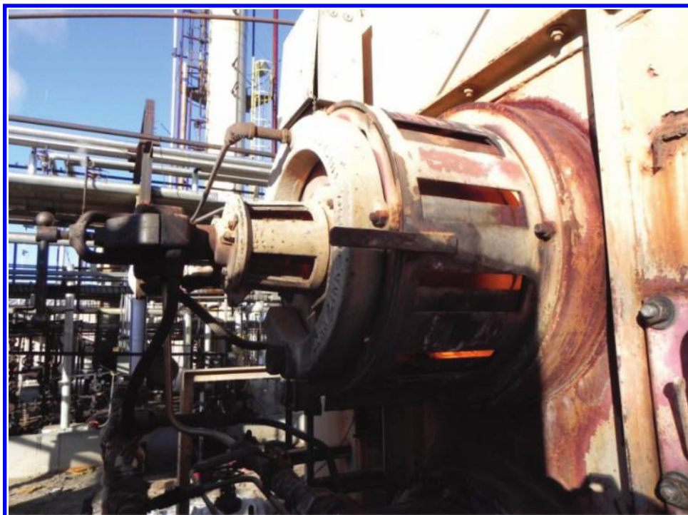
FIGURE 2.16 Typical rotary-type air registers.
