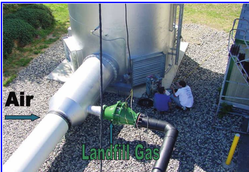
FIGURE 13.16 ZULE static mixing chamber.
