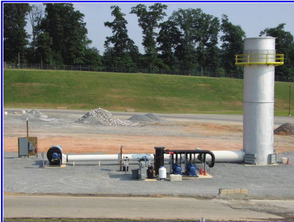
FIGURE 13.15 Zink Ultra Low Emission (ZULE®) enclosed flare.
