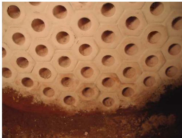
FIGURE 15.18 Boiler ferrules—after repair.
