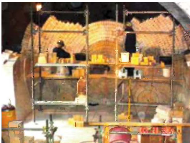
FIGURE 5.10 Example of labor-intensive brick installation.
