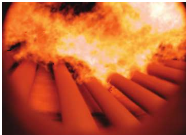
FIGURE 13.53 Flame impingement.
