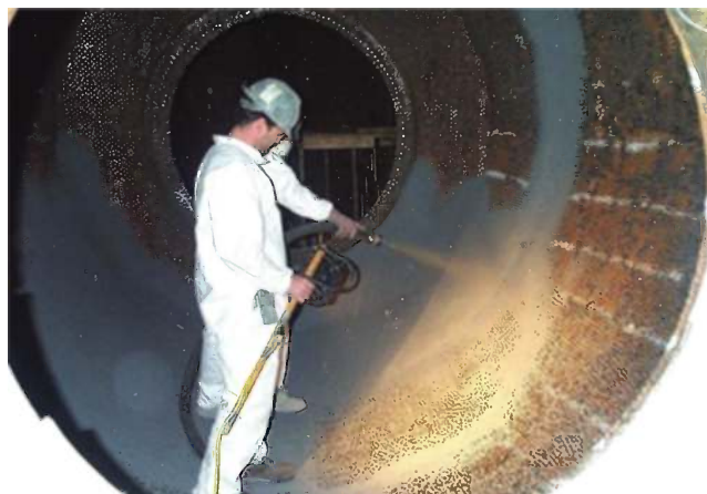
FIGURE 5.36 Example of vessel having refractory spray installed.
