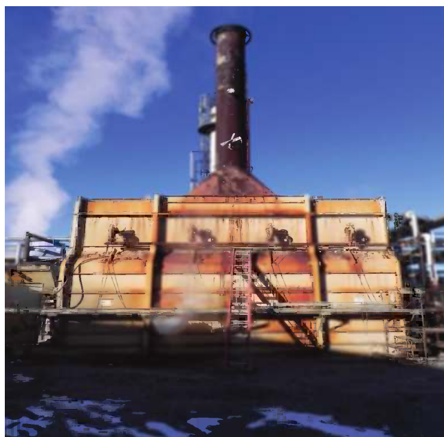
FIGURE 12.41 Heater casing oxidation.
