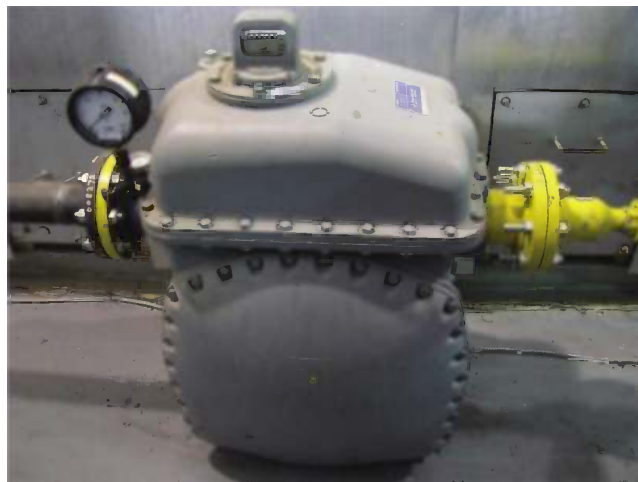
FIGURE 7.21 Positive displacement meter.
