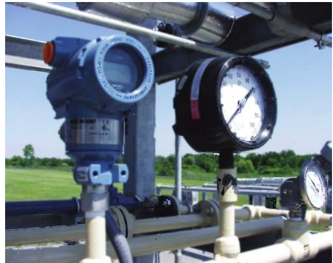
FIGURE 2.19 Pressure transmitter (left) and pressure gage (right).
