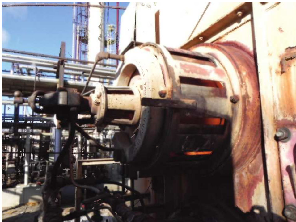
FIGURE 11.111 Typical rotary-type air registers.
