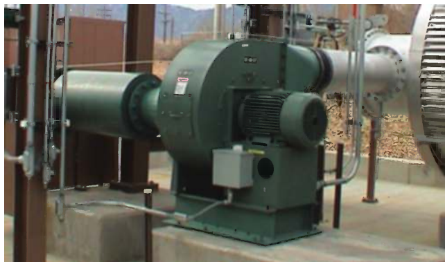
FIGURE 3.7 An arrangement 4 fan.
