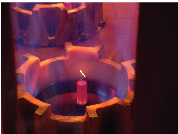
FIGURE 11.137 Operating pilot with flame rod.
