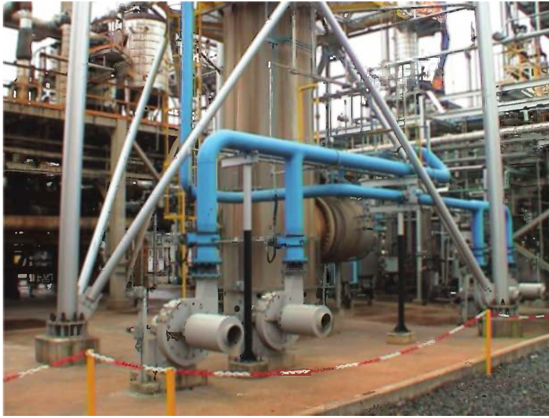
FIGURE 3.13 One primary and one backup fan in the field with ducting.
