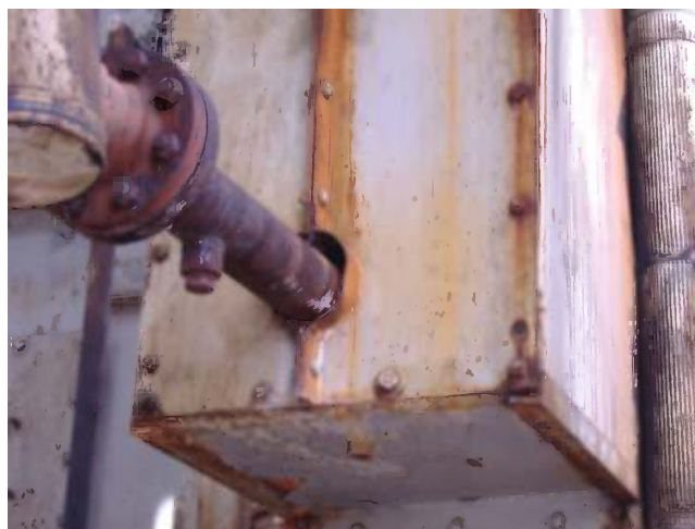
FIGURE 12.14 Air leakage around process tube.
