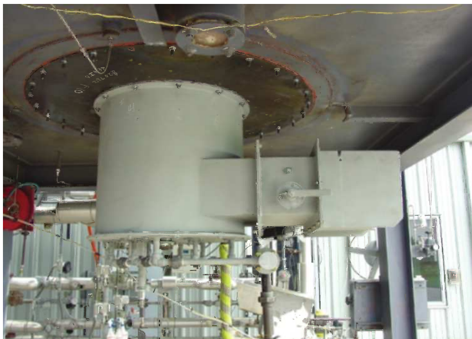
FIGURE 11.113 Integral plenum box with inlet air damper and muffler.
