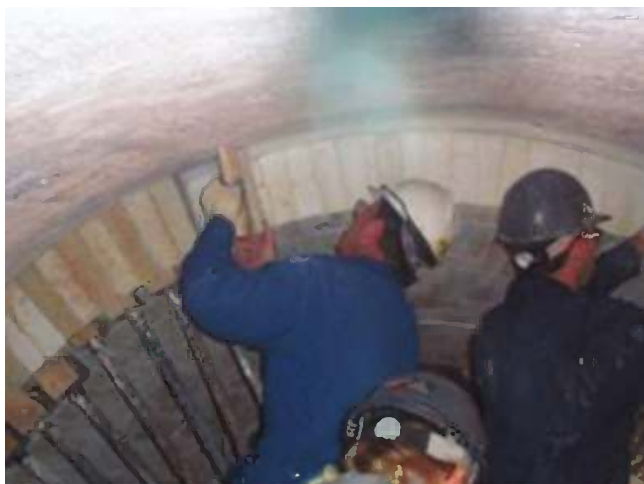
FIGURE 5.12 Use of pogo sticks to ensure brick is properly seated.
