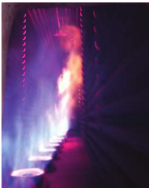
FIGURE 13.33 Flames short of air and impinging on tubes.
