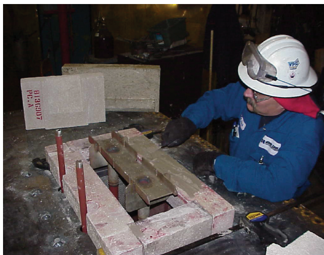
FIGURE 11.10 Applying mortar to burner tile.
