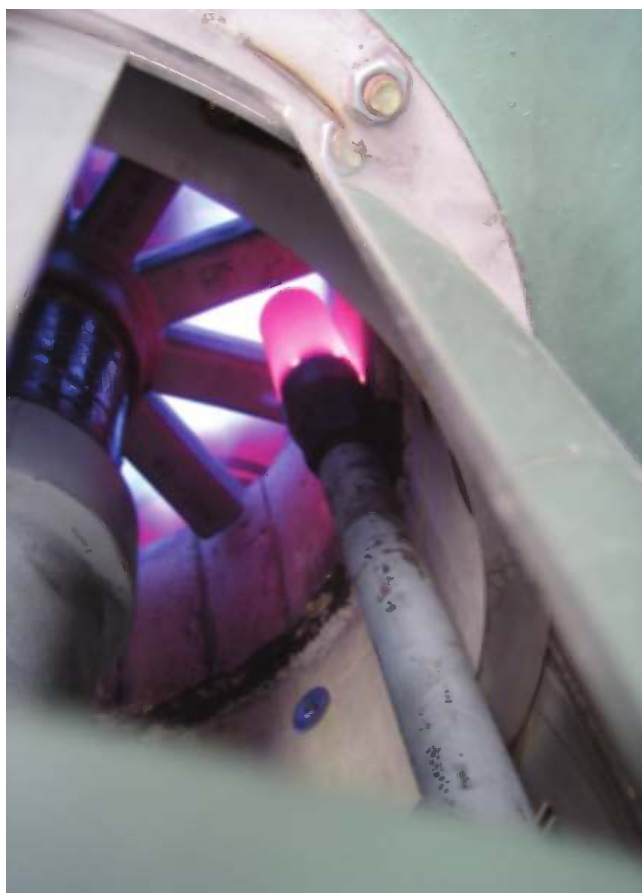
FIGURE 11.131 Pilot shield glowing in normal operation.
