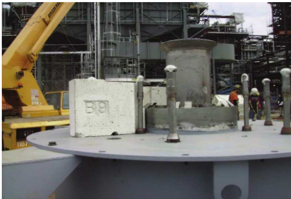
FIGURE 11.12 Tile with groove-clearing bolt heads.
