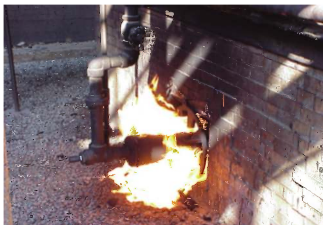
FIGURE 12.1 Flames outside the heater.
