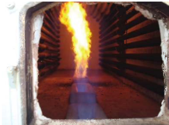
FIGURE 12.35 Uneven flame patterns.
