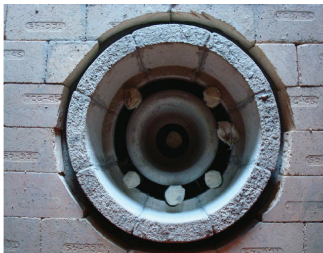
FIGURE 11.11 Gas tips protected with masking tape during installation.
