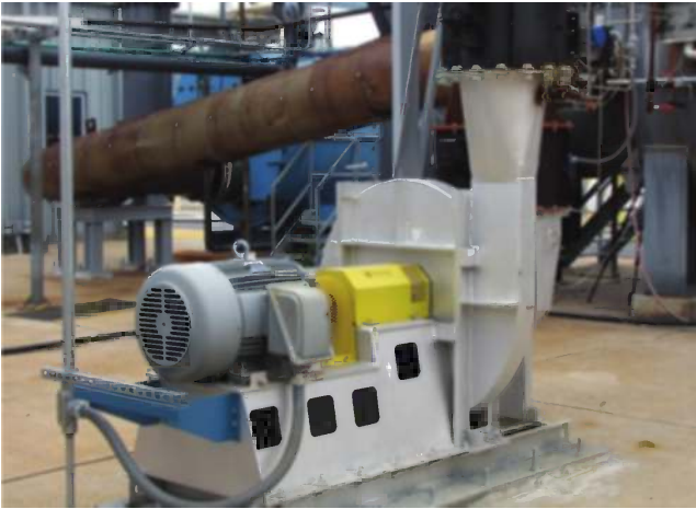
FIGURE 3.1 A centrifugal fan.
