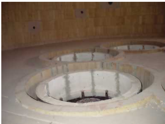
FIGURE 5.11 Firebricks cut and installed in a circular pattern.
