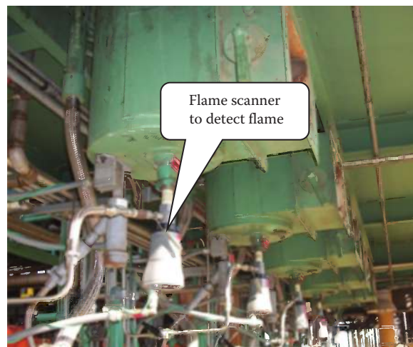
FIGURE 11.42 Burners with flame scanners.
