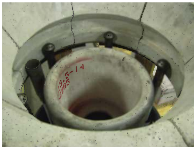
FIGURE 13.55 Combination burner with Regen (oil) tile.
