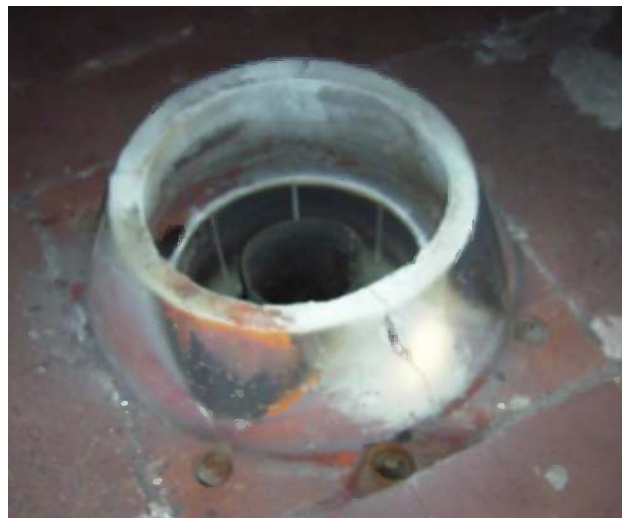
FIGURE 11.85 Tile with large cracks should be replaced.
