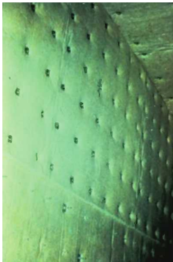
FIGURE 5.17 Photograph of installed ceramic refractory.
