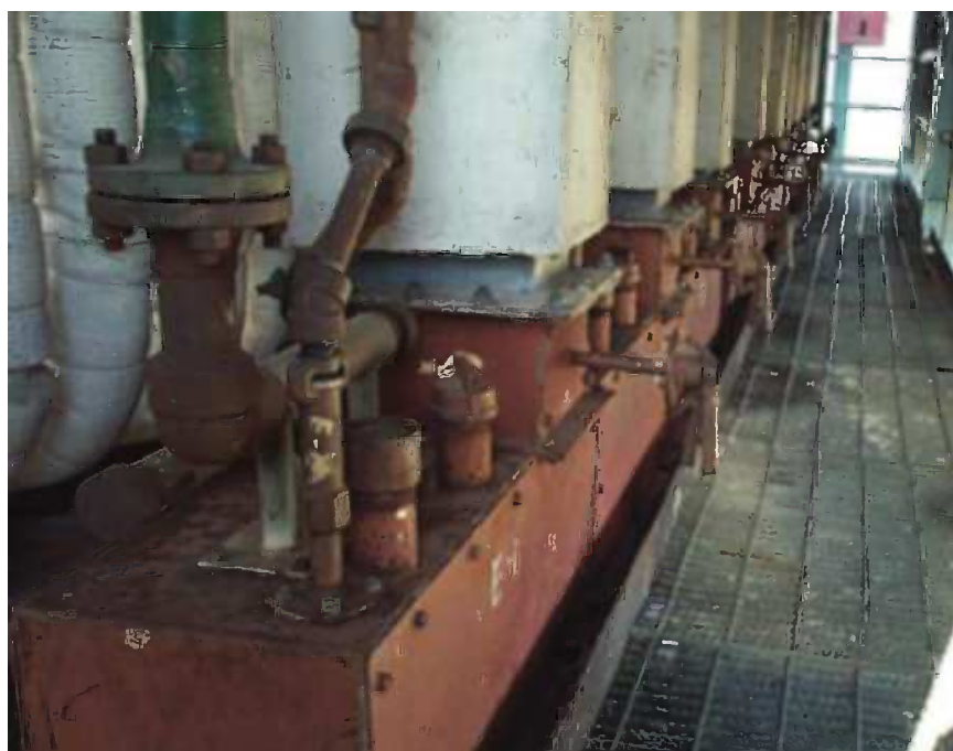
FIGURE 11.28 Down-fired burners located on top of the heater.
