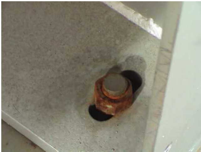
FIGURE 15.9 Sliding anchor bolt.
