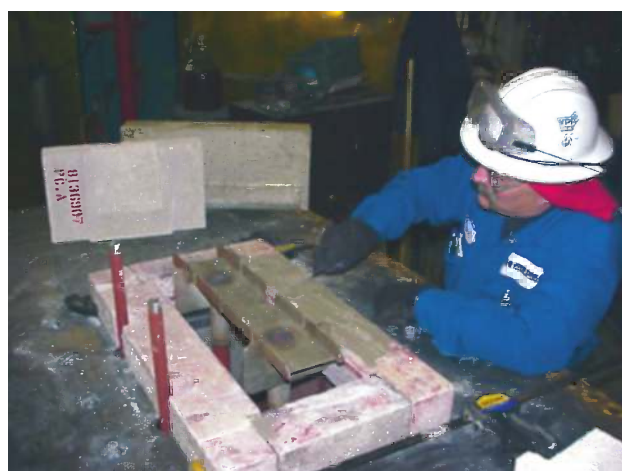
FIGURE 11.86 Applying a thin layer of mortar.
