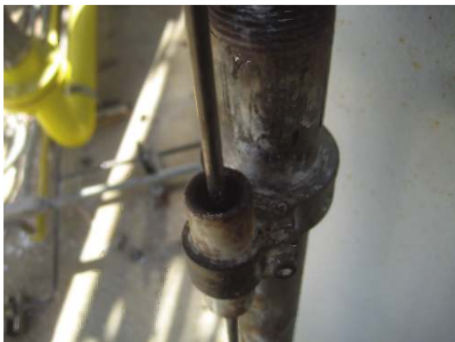
FIGURE 15.7 Dirty pilot ceramic insulator.
