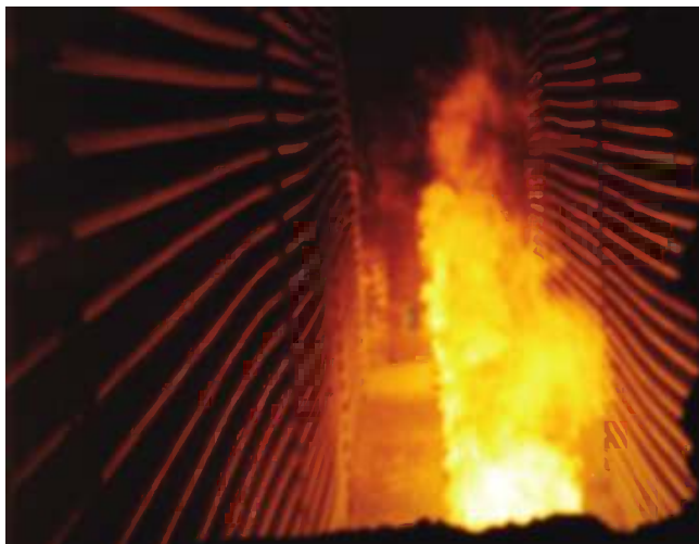
FIGURE 13.59 Flame impingement.
