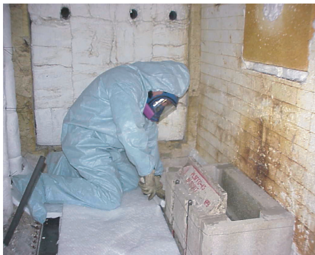
FIGURE 11.88 Final tile installation.
