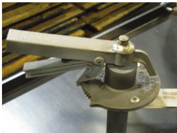
FIGURE 11.101 Locking air control handle with 18 positions.
