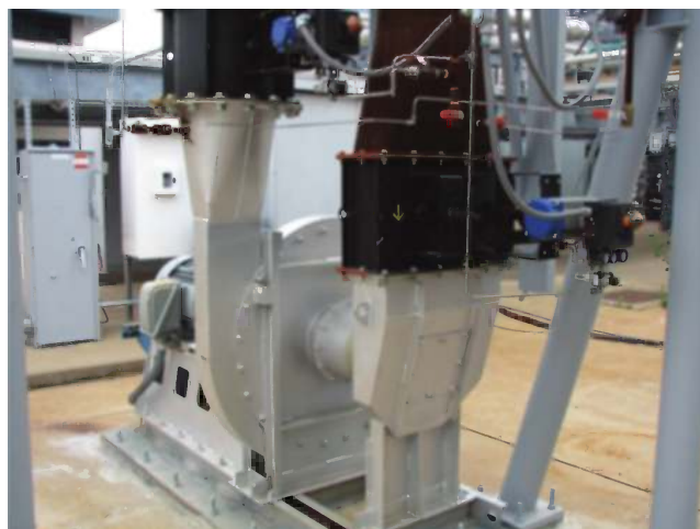
FIGURE 3.17 Centrifugal fan with inlet and outlet dampers.
