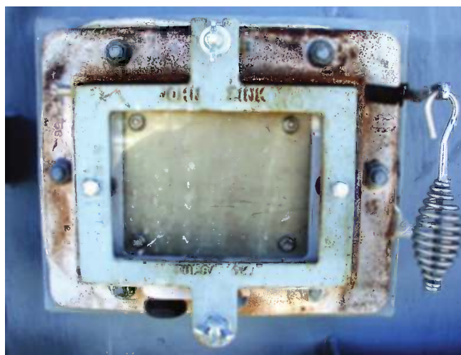
FIGURE 1.8 Viewport with shutter. (From Baukal, C.E., Industrial Combustion Pollution and Control , Fig. 11.15, Marcel Dekker, New York, 2004.)
