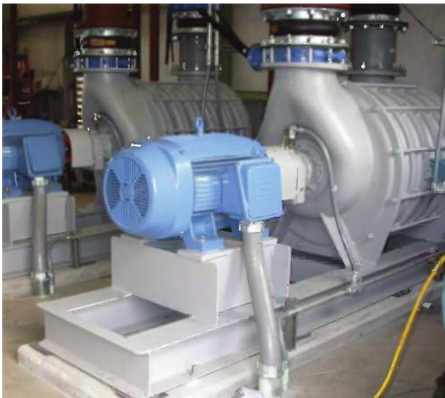
FIGURE 3.5 A multistage high-speed centrifugal blower for a landfill application.
