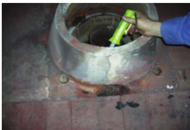
FIGURE 11.84 Small cracks can be repaired.
