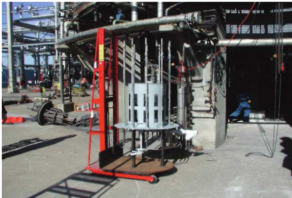
FIGURE 11.16 Lifting device for burner installation.
