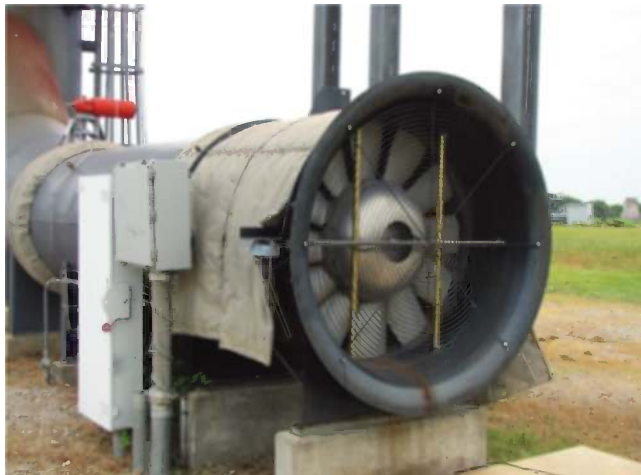
FIGURE 3.3 A vane axial fan.
