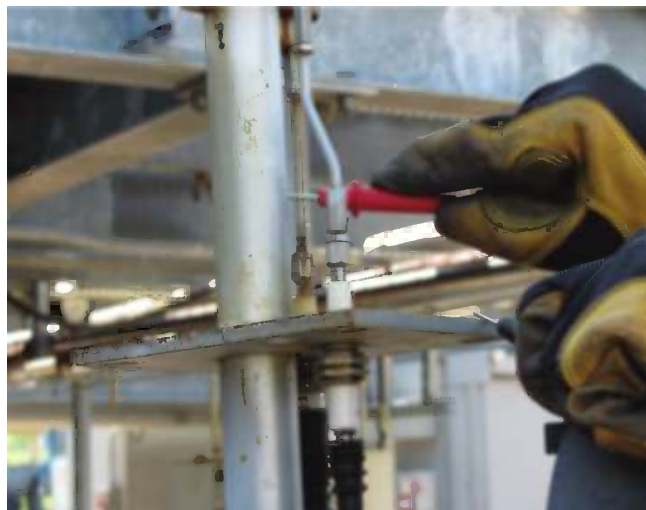
FIGURE 13.13 Connecting test probes for flame voltage.
