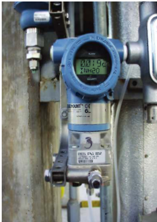
FIGURE 12.9 Draft transmitter.
