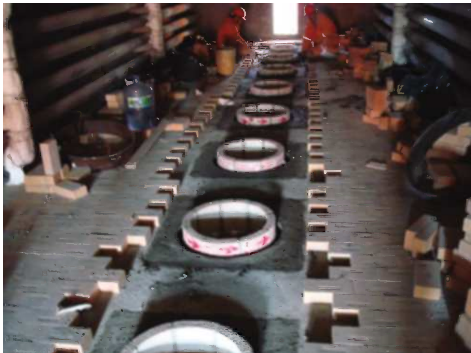
FIGURE 11.9 Burner tiles with mortared joints.
