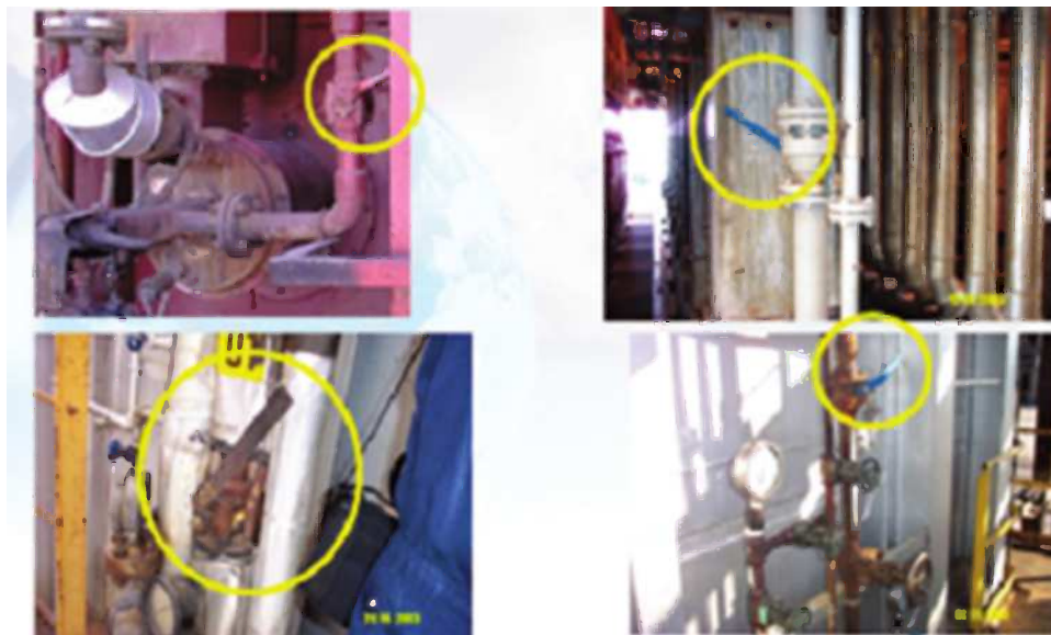
FIGURE 12.40 Examples of pinched block valves.
