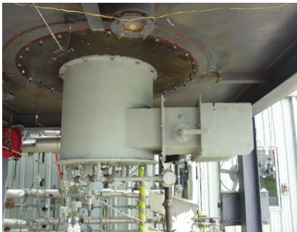
FIGURE 11.21 P-box-type burner with an integral plenum.
