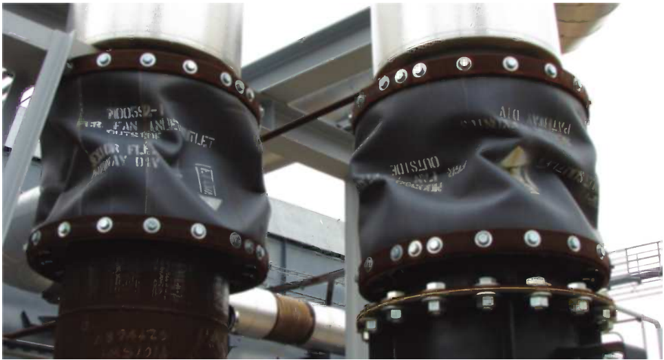
FIGURE 3.26 Inlet and outlet expansion joints for vibration isolation of ducting.
