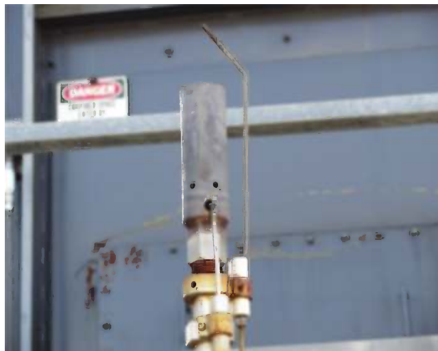
FIGURE 13.6 ST-1SE-FR pilot which includes a flame rod.
