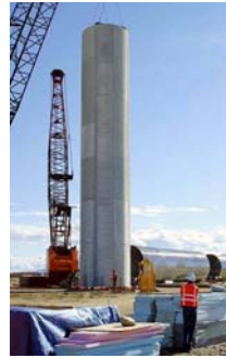
A silo liner being lifted into place for installation into a missile silo at a launch complex under
