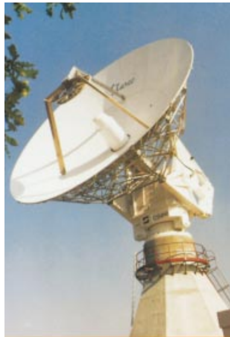
Figure 12-17: A typical, but large telemetry reception antenna.
