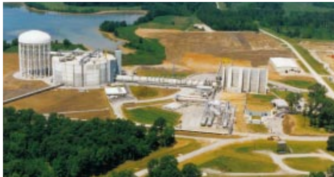
Figure 15-19: A large rocket test facility capable of simulated altitudes of up to 33,000 m.
