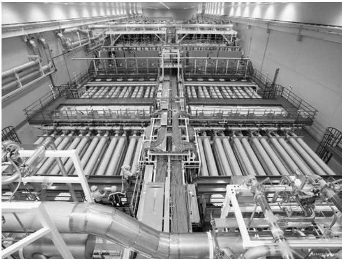
FIGURE 13.5 One of the two laser bays showing 24 beamlines in NIF.
