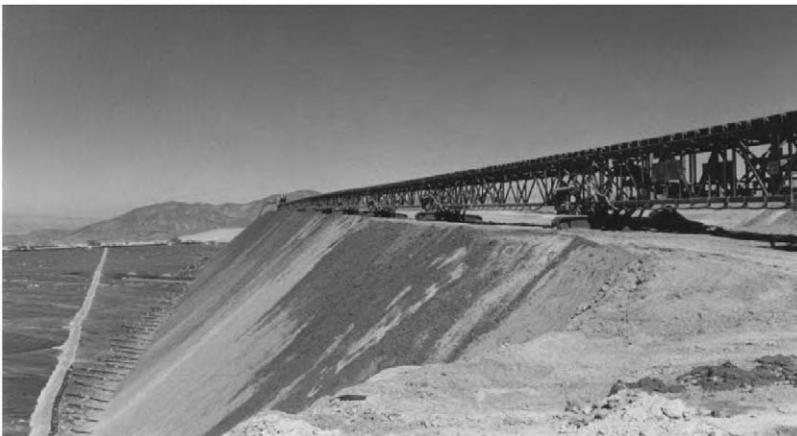
Fig. 4. Rahco stacker building a 12m lift by tripping the ore over the advancing edge. The stacker can climb ramps and turn sharply to fit project requirements.
