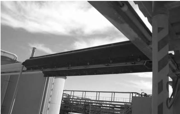
Fig. 8. Secondary containment for pipelines.
