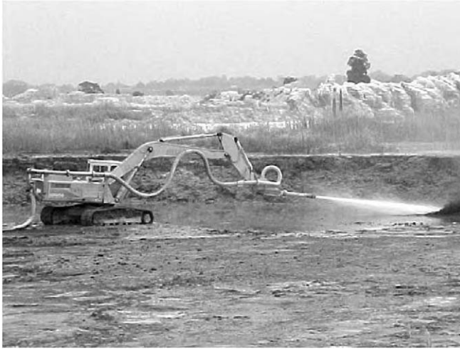
Fig. 1. Excavator-mounted monitor gun.
