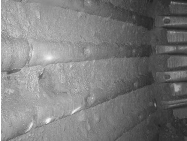
Fig. 5. Packed shell lifters after liner change-out in a 10.4 m (34') SAG mill.
