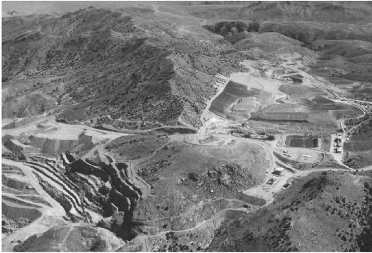
Fig. 2. Heap leach installation at Mineral Ridge, Nevada (Golden Phoenix Minerals, Inc.). The open pit mine is shown on the left. On the right is a 2 Mt heap of crushed, conveyor-stacked ore placed on a plastic-lined leach pad. Pregnant and barren solution storage ponds are located downslope from the heap. Buildings include process plant, laboratory, maintenance shop and administration offices. (Photograph courtesy of Tom Nimsic, American Au/Ag Associates).
