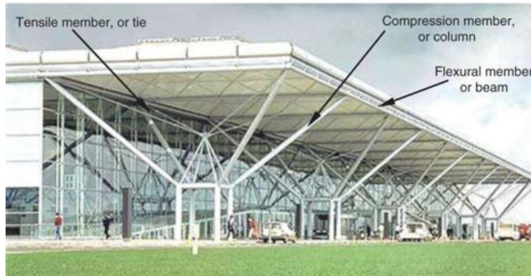
Modes of loading. (Image of Stansted Airport courtesy of Norman Foster and Partners, London, UK)
