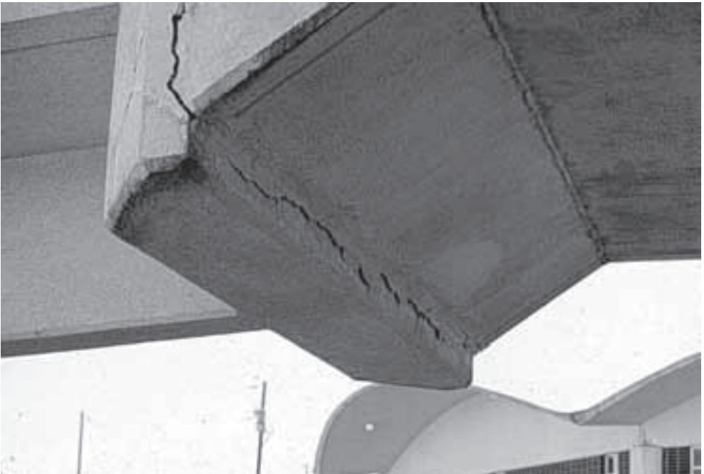
FIGURE 8.3 Structural damage caused by expansive clay soil.
