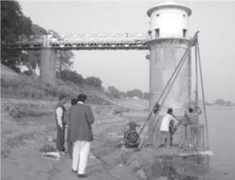
FIGURE 10.3 Wash boring method.
