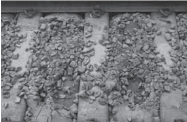
FIGURE 14.12 Migration of fines from subgrade into ballast.
