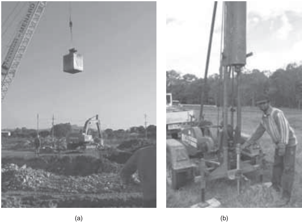
FIGURE 1.9 (a) Dynamic compaction and (b) JCU heavy dynamic cone penetration test rig.
