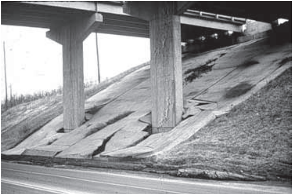
FIGURE 8.9 Slope movement under bridge and against supports.
