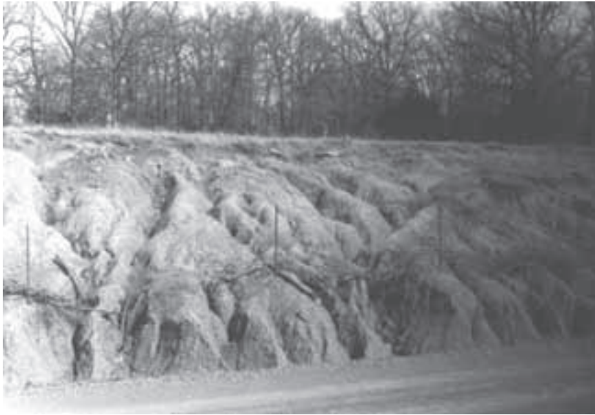
FIGURE 9.1 Slope with dispersive clay and surface reaction erosion.
