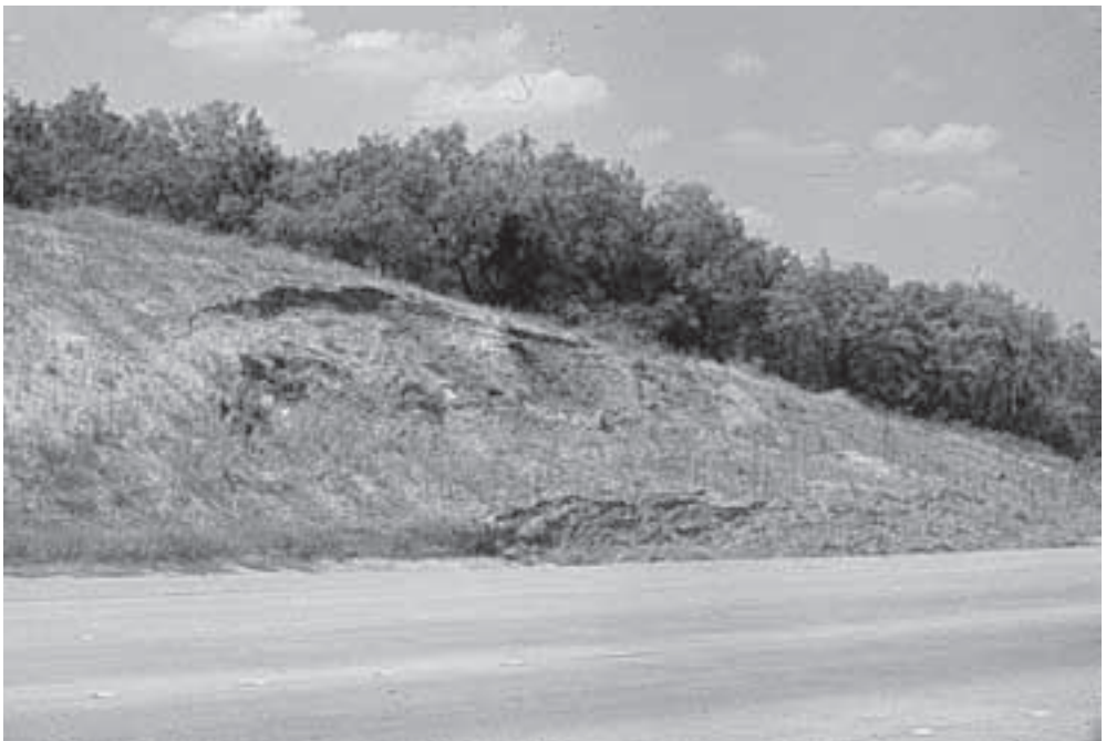
FIGURE 8.10 Typical slope failure in expansive clay.
