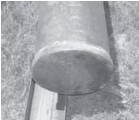
FIGURE 5.3 Closed end of a steel pipe pile.
