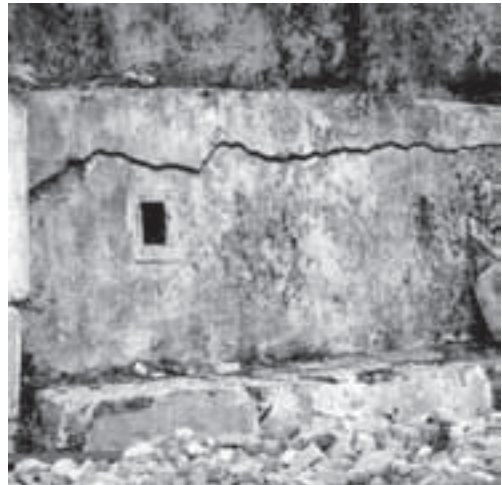
FIGURE 6.27 Cracks on retaining wall due to excessive settlement of foundation.
