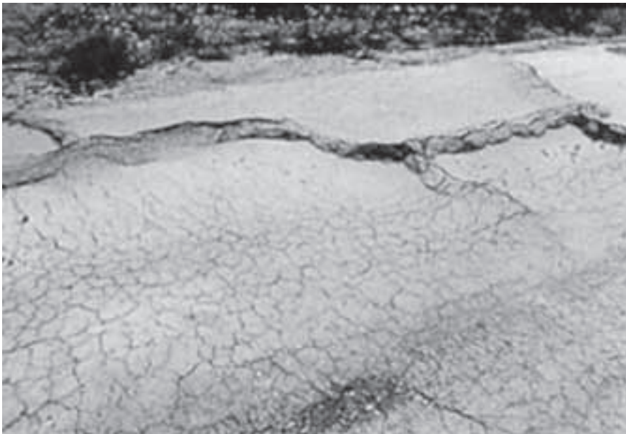
FIGURE 9.4 Results of sulfate-induced heave on roadway.
