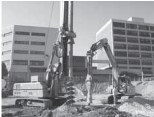
FIGURE 5.8 Construction of a geopier.
