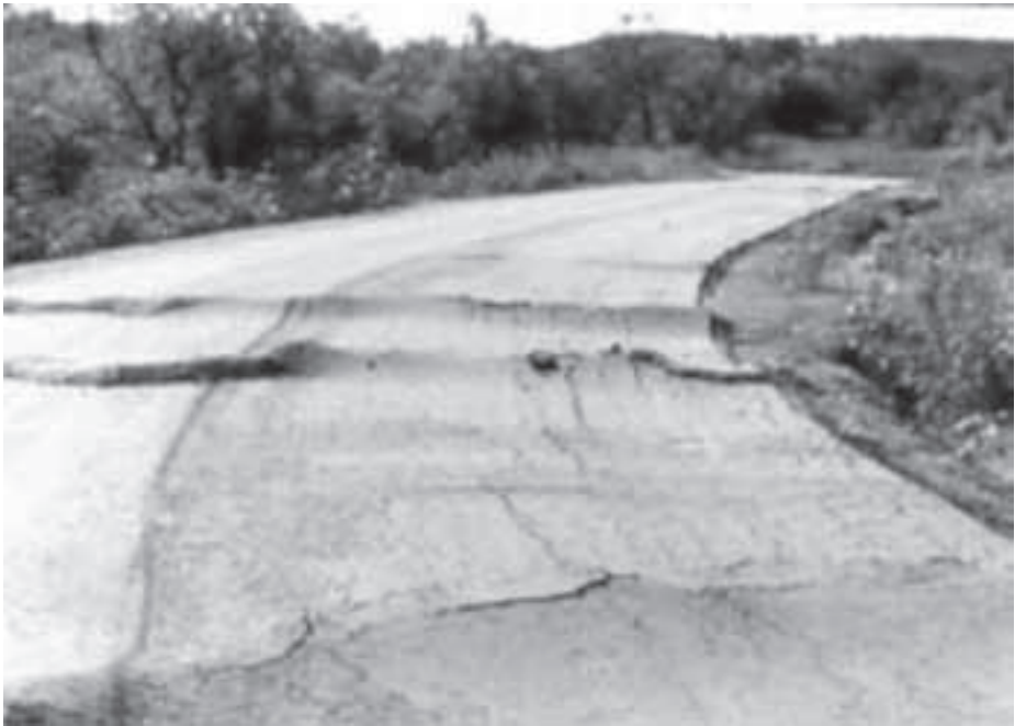
FIGURE 9.5 Buckling of roadway by sulfate-induced heave.
