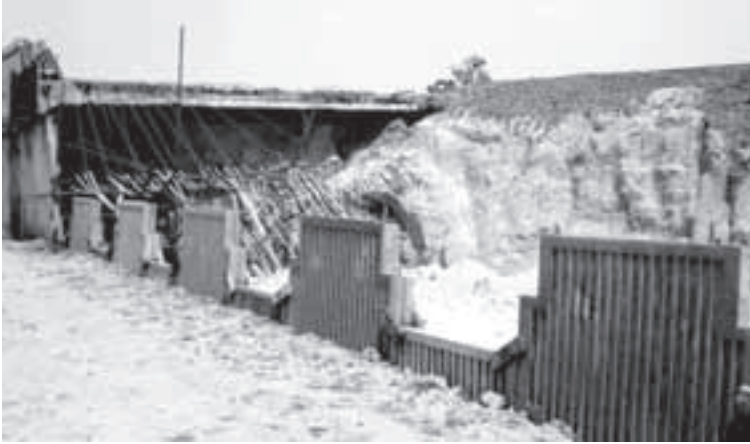
FIGURE 6.29 Failure of mechanically stabilized retaining wall due to rupture of ties.
