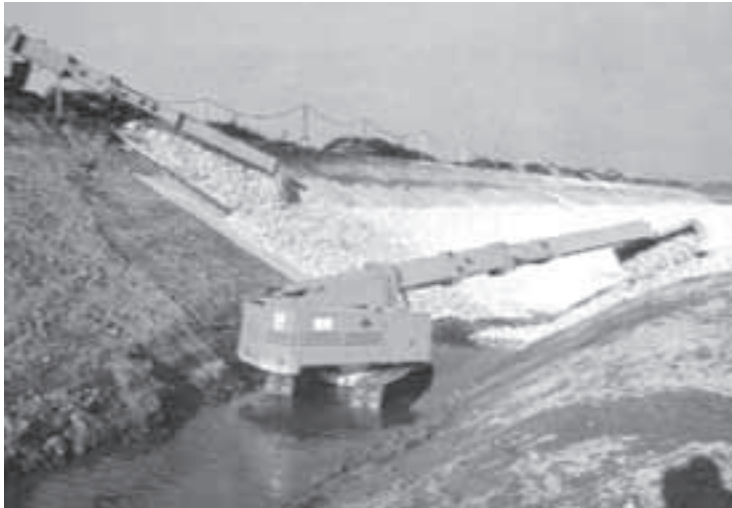
FIGURE 12.8 Geotextile filters in stream bank protection.
