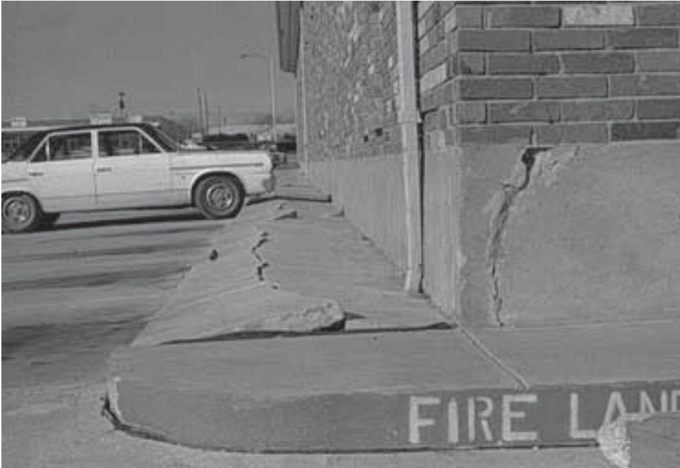
FIGURE 8.1 Typical distress caused by expansive clays.
