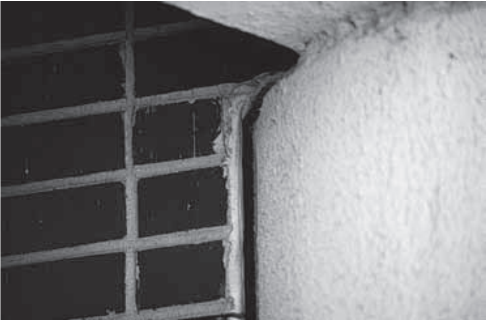
FIGURE 8.2 Differential movement between wall and column caused by expansive clay soil.
