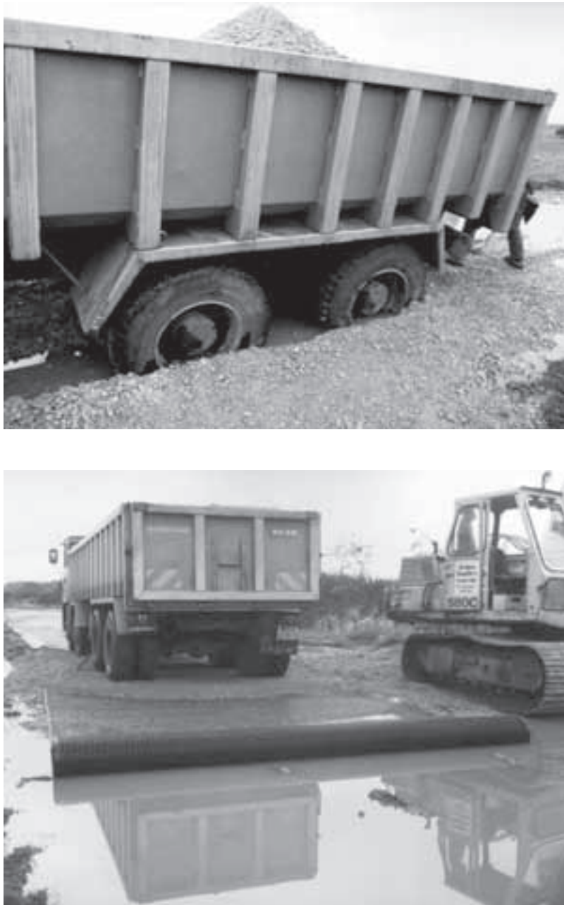
FIGURE 12.18 Road before (top) and after (bottom) reinforcement with geosynthetics.
