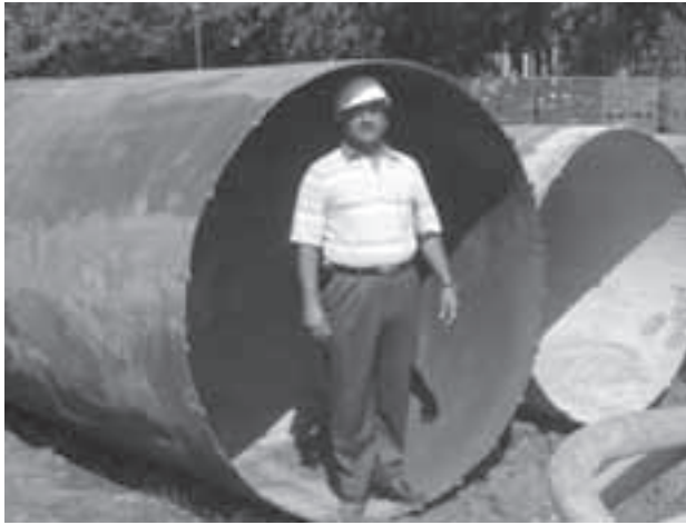
FIGURE 5.7 Steel casing for construction of drilled shafts.
