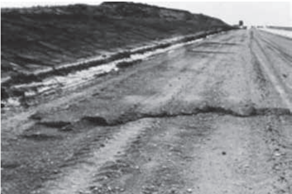
FIGURE 9.6 Sulfate-induced heave in interstate highway subgrade.
