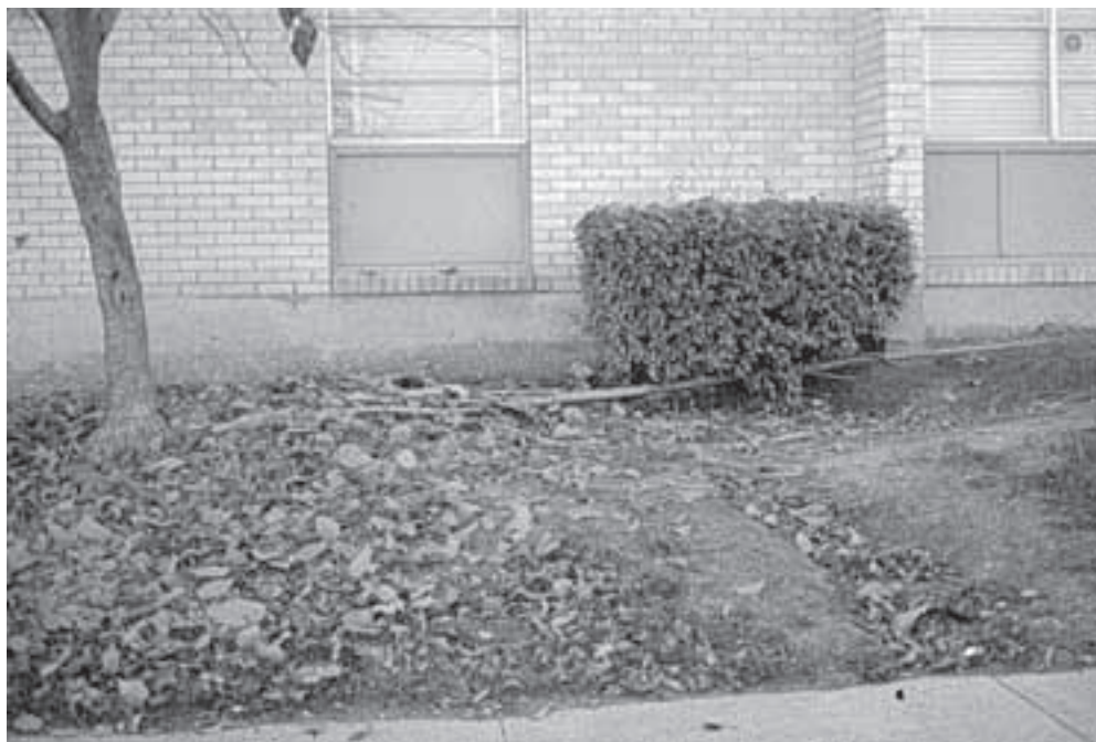
FIGURE 8.11 Typical tree root, bush, and poor exposure of building exterior.
