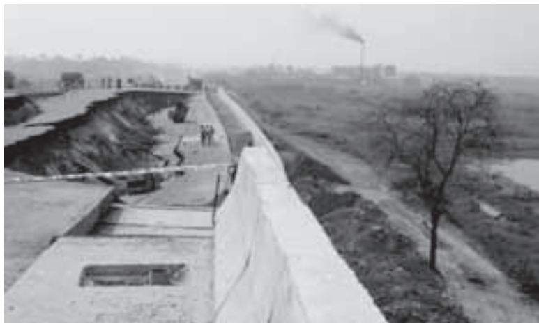
FIGURE 6.28 Deep-seated rotational failure of wall in soft clay.
