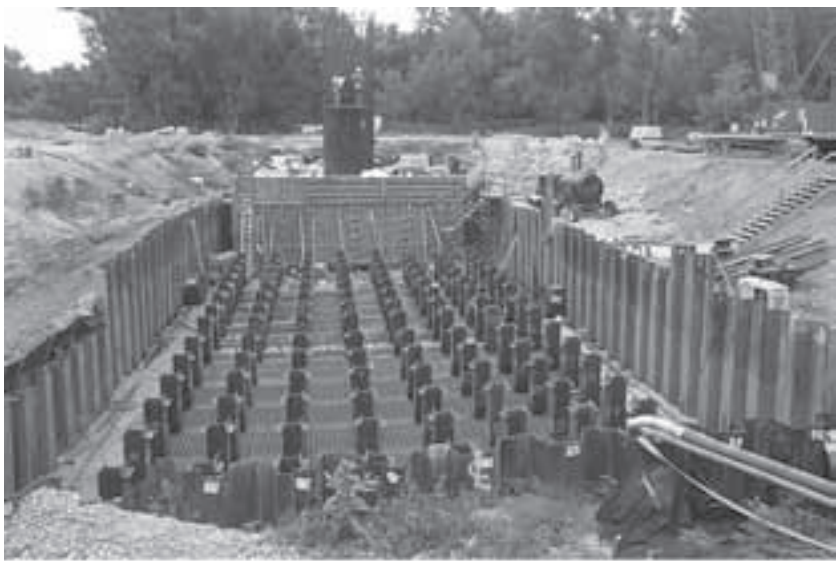
FIGURE 5.46 A group of steel H-piles for construction of a bridge pier (before construction of the pile cap).
