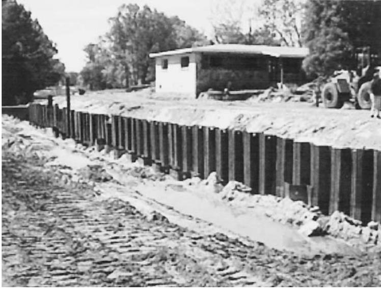
**FIGURE 15.1** A flexible retaining wall under construction.
