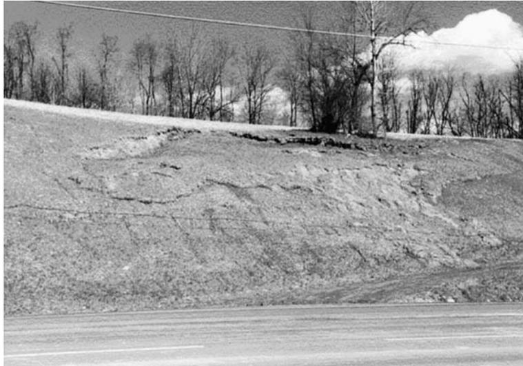
**FIGURE 16.1** Slope failure near a roadway. (Courtesy of Todd Mooney.)
