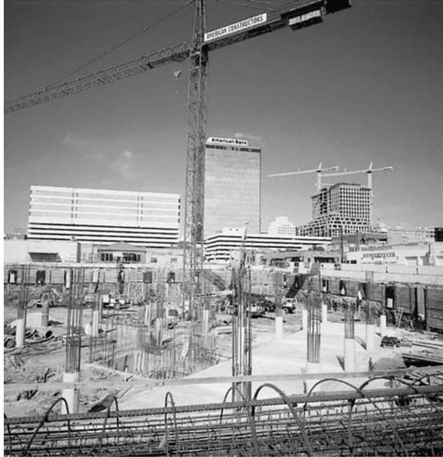
**FIGURE 13.1** Concrete piles used for the foundation of a skyscraper. (© Fritz Henle/Photo Researchers.)
