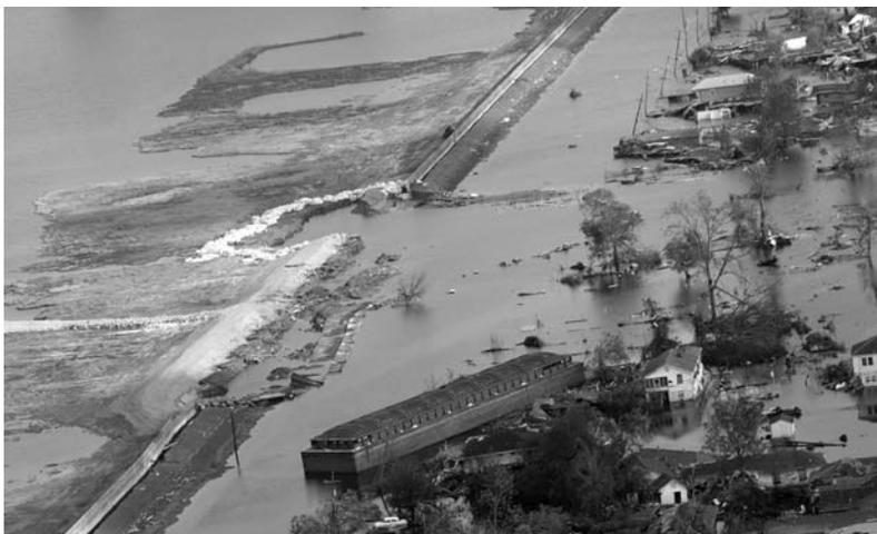
**FIGURE 5.1** Failure of a section of a levee from Hurricane Katrina.
