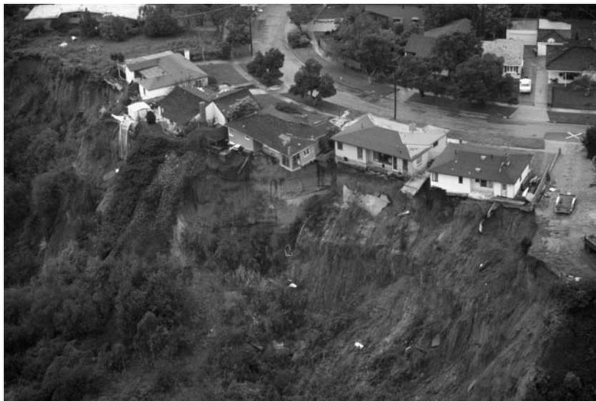
**FIGURE 10.1** Shear failure of soil under several homes. (©Vince Streatano/Corbis.)
