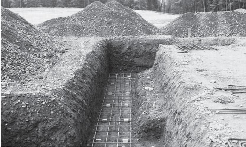
**FIGURE 12.1** Construction of a shallow foundation.
