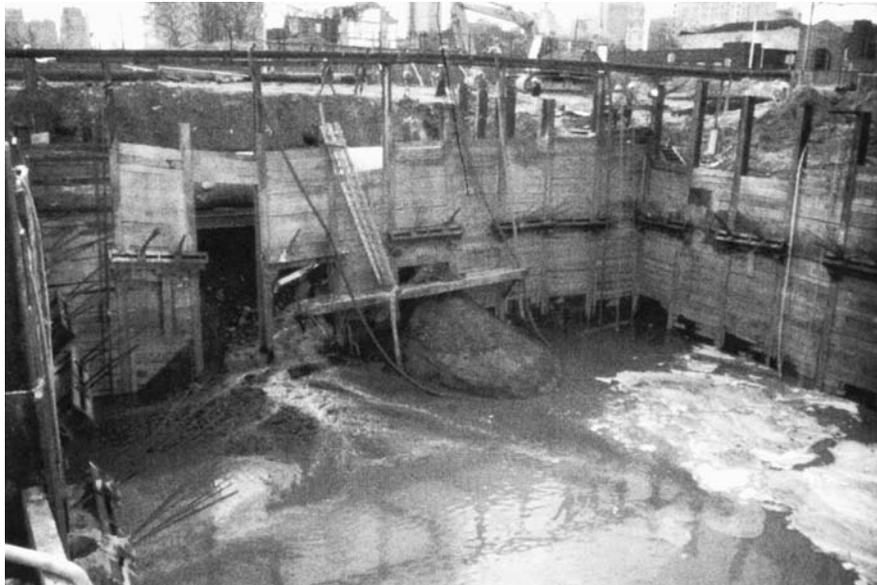
**FIGURE 14.1** Damage to a braced excavation by seepage forces. (Courtesy of George Tamaro, Mueser Rutledge Consulting Engineers.)
